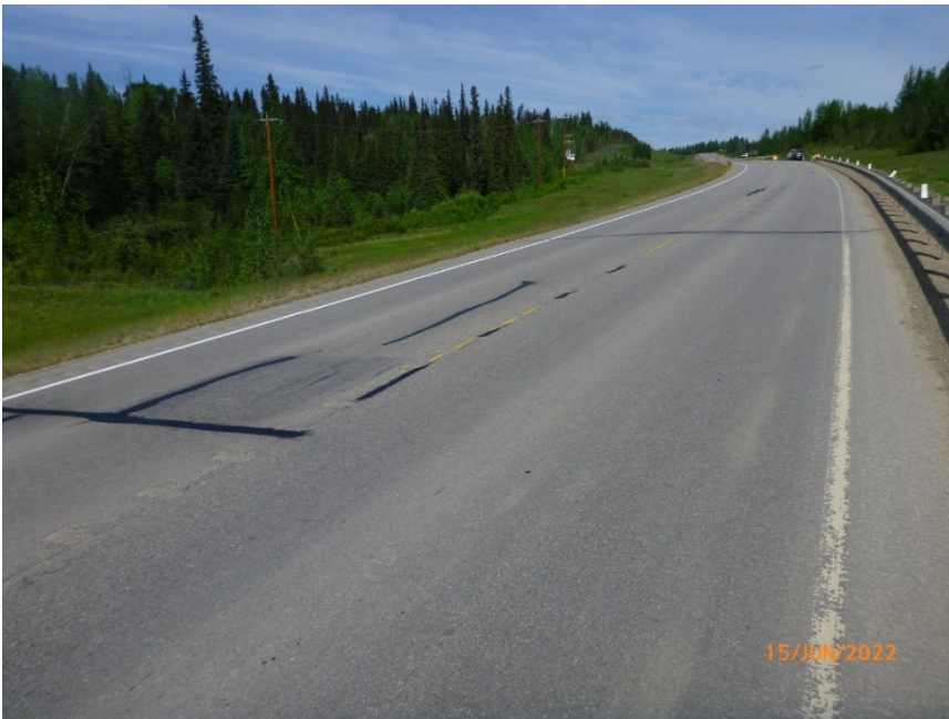
Photo 6 Minor cracking in pavement surface of Hwy 40:38 at GP038-II site. Photo taken June 15, 2022, facing northwest.
