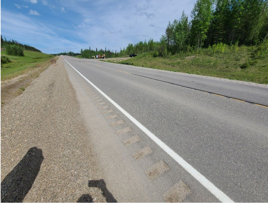
Photo 2 Settlement in pavement surface of Hwy 40:38 at GP038-I site at WP213. As well as rill erosion along south side of highway embankment. Photo taken June 15, 2022, facing southeast.
