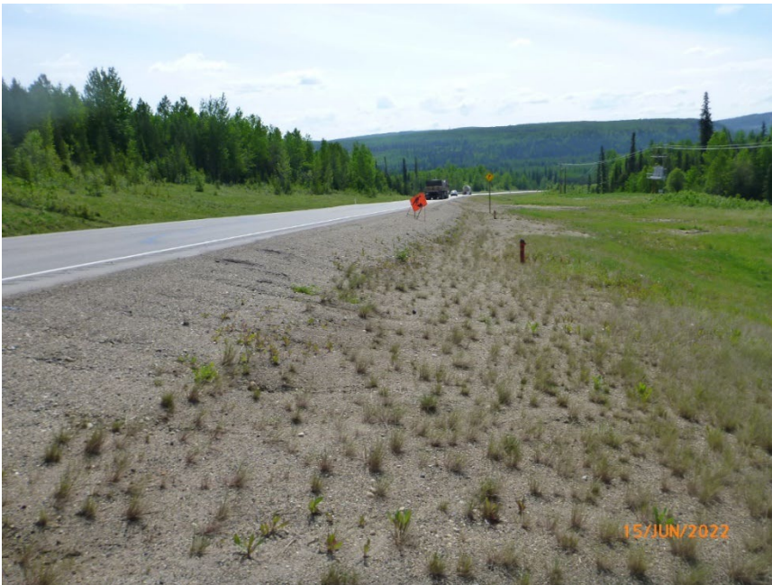
Photo 2 Settlement in pavement surface of Hwy 40:38 at GP038-I site at WP213. As well as rill erosion along south side of highway embankment. Photo taken June 15, 2022, facing southeast.
