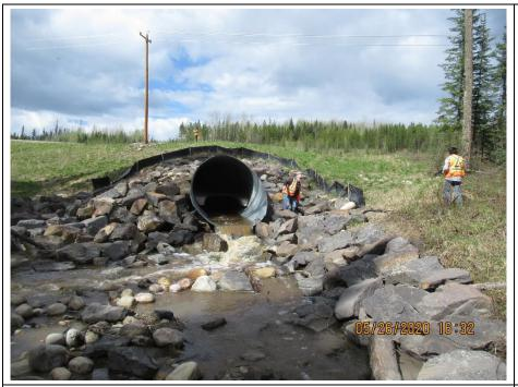
Photo 3. Looking north at the 2.43 m diameter SPCSP outlet and riprap.
