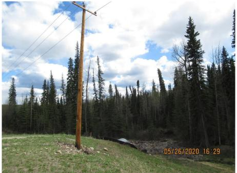
Photo 10. Looking southeast at new power pole that was installed on toe berm near culvert alignment.
