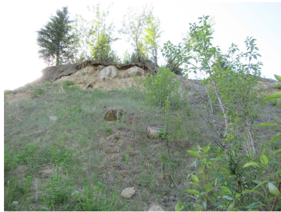
Photo 9. Looking west up at hanging boulders that will eventually fall into ditch or highway.
