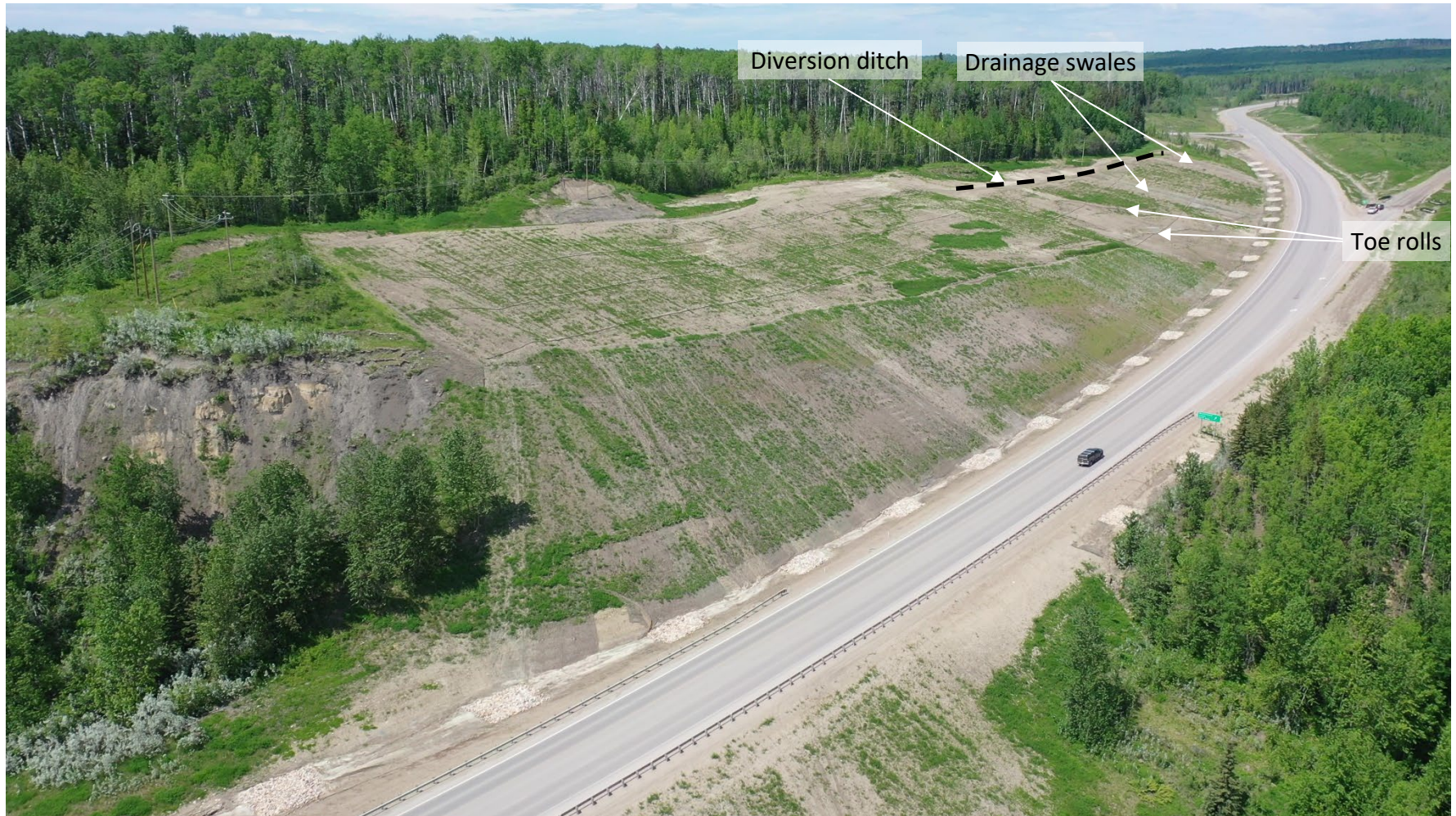
Photo 2 Overview of GP044 site on Hwy 40:40. Photo taken June 15, 2022, facing southwest from southern site limit.
