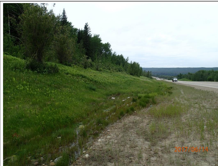
Photo 3. Looking northwest along the NBL ditch.
