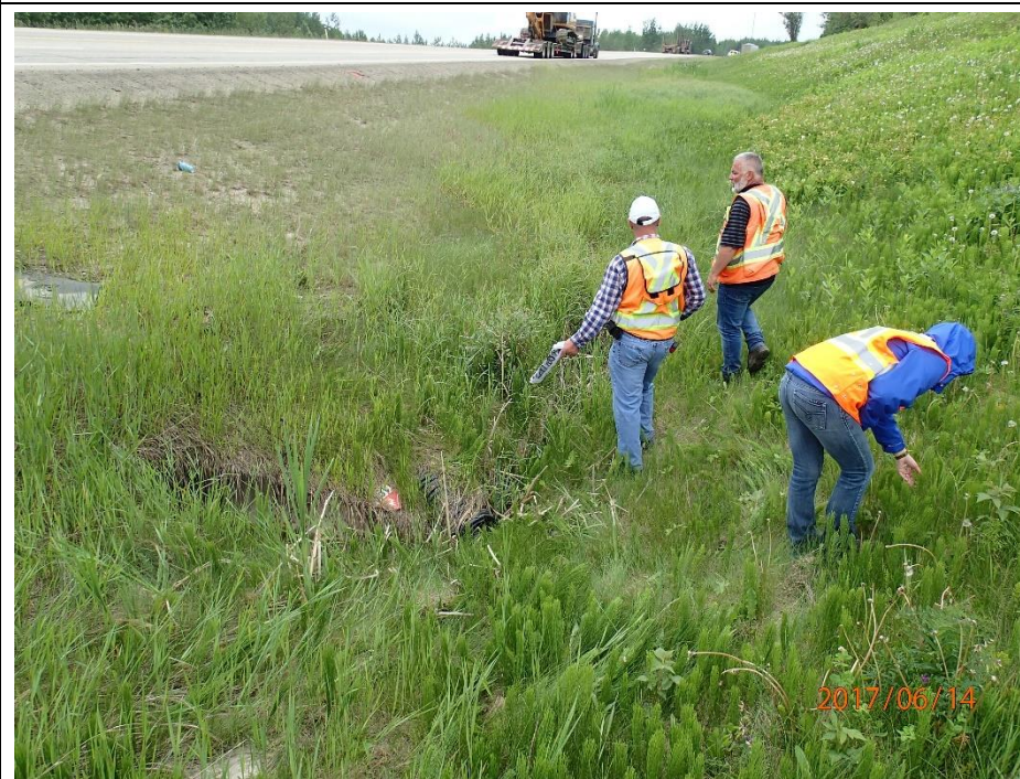
Photo 10. Looking southeast at km 25.71 at west ditch and culvert inlet.
