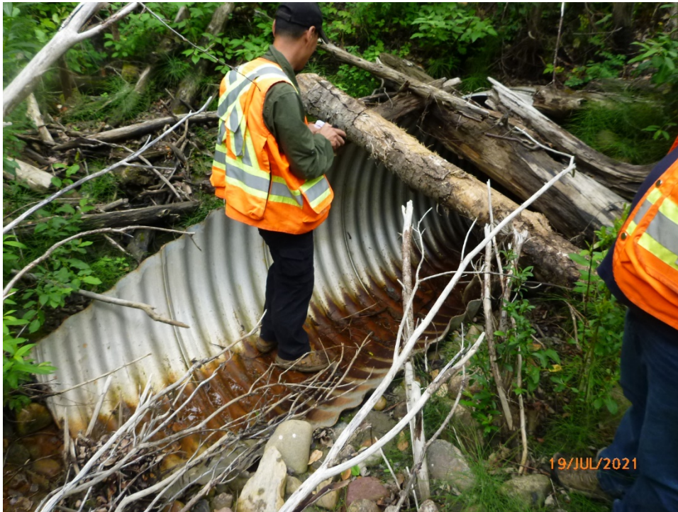
Photo 6 Inlet of 1200 mm diameter CSP culvert. Photo taken July 19, 2021 facing southeast.
