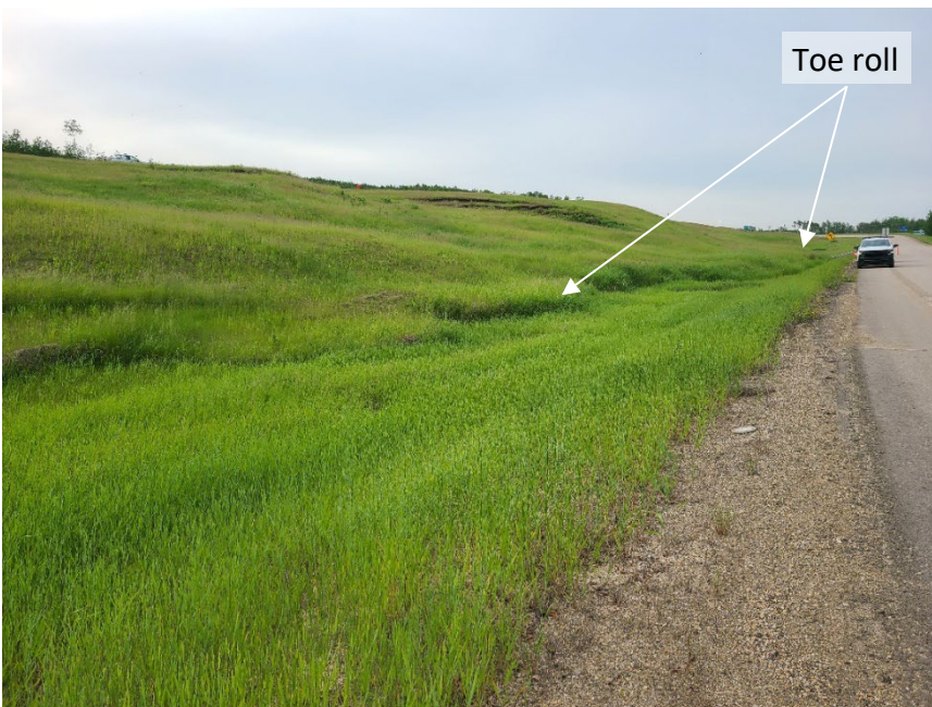
Photo 2 Toe roll at WP079 along/in east ditch of southbound lanes of Hwy 43:04. Photo taken June 16, 2022, facing southeast.
