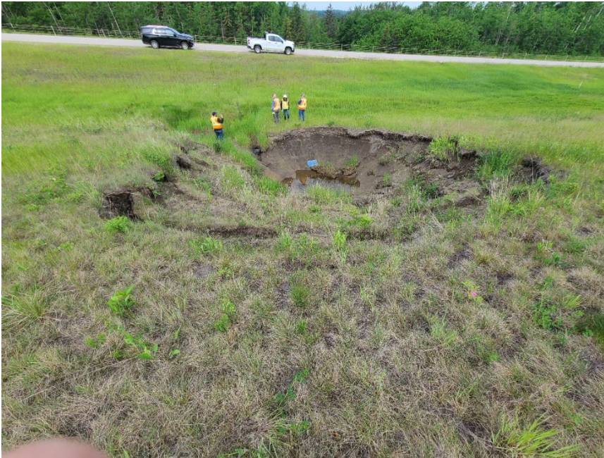
Photo 6 Crest of erosion gully at 0.9-m diameter SWSP culvert outlet at WP076. Note reference/survey stakes with flagging (circled in white) placed 2.0 m upslope of erosion gully to monitor retrogression. Photo taken June 16, 2022, facing south.
