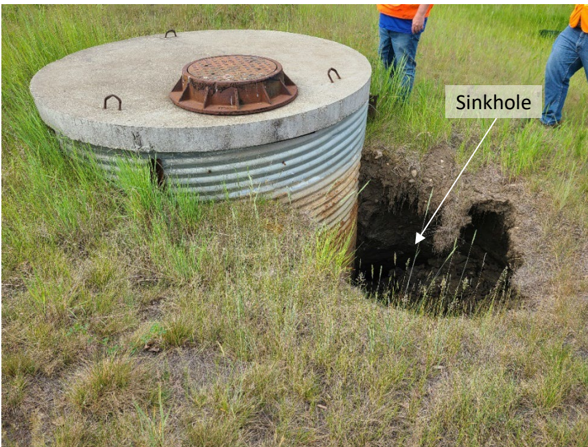
Photo 12 Sinkhole at WP226 next to inlet of CSP drainage gallery in median backslope above of southbound lanes of Hwy 43:04. Photo taken June 16, 2022, facing west.
