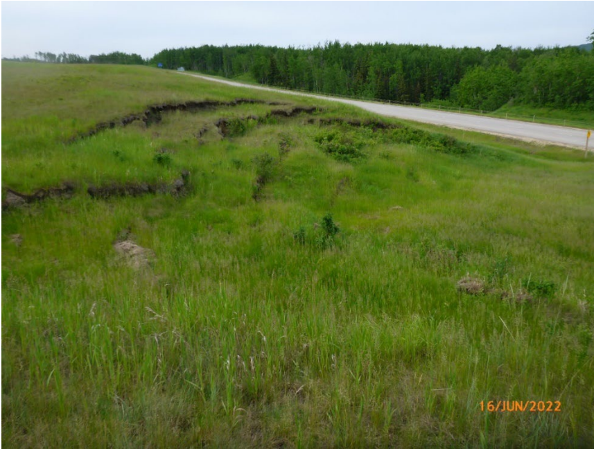
Photo 2 Toe roll at WP079 along/in east ditch of southbound lanes of Hwy 43:04. Photo taken June 16, 2022, facing southeast.
