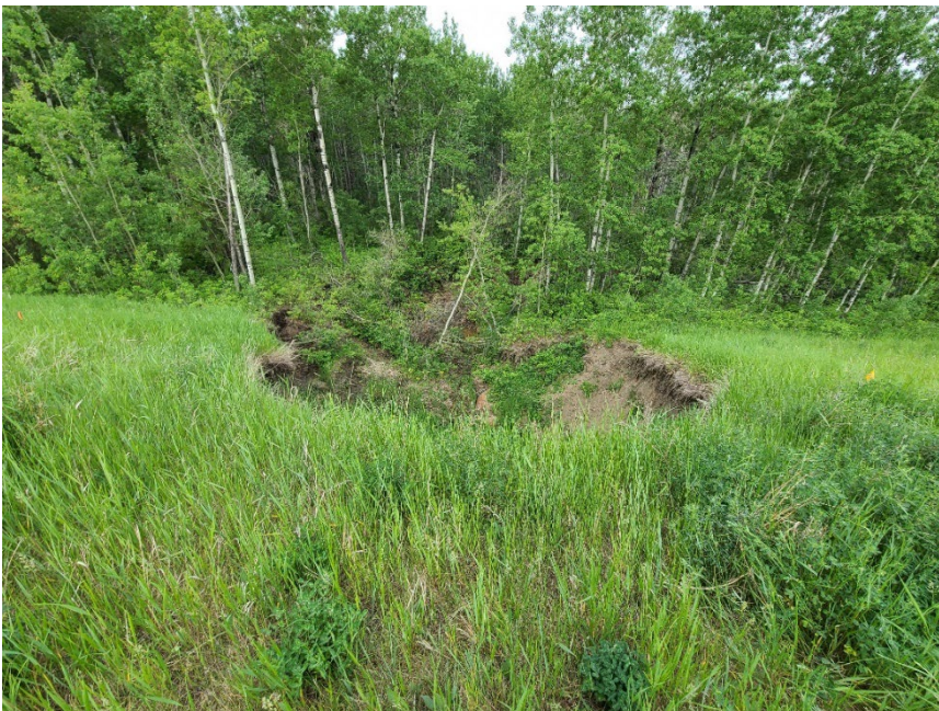
Photo 8 Erosion gully at 1.2-m diameter CSP culvert outlet at WP227. Photo taken June 16, 2022, facing west.
