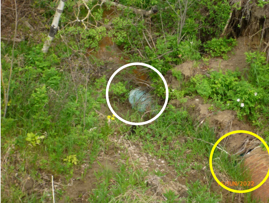
Photo 12 Sinkhole at WP226 next to inlet of CSP drainage gallery in median backslope above of southbound lanes of Hwy 43:04. Photo taken June 16, 2022, facing west.
