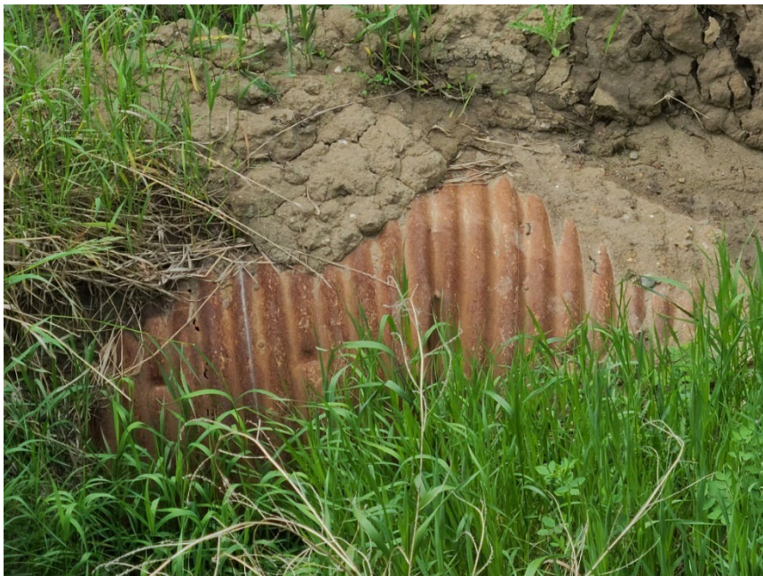
Photo 10 Outlet of 1.2-m diameter culvert corroded with holes at WP227. Photo taken June 16, 2022, facing south.
