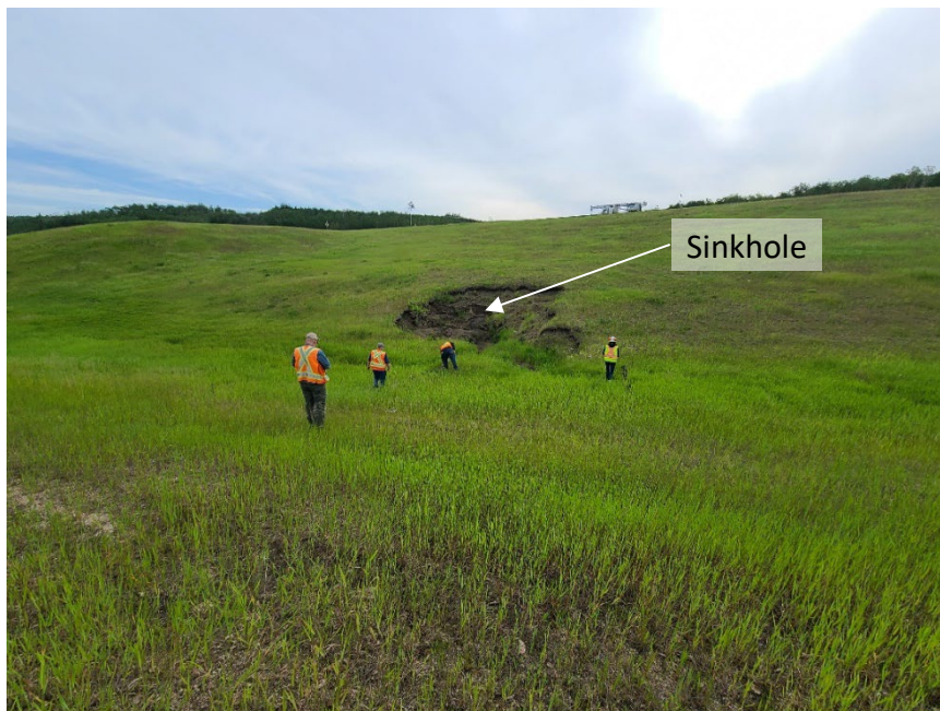
Photo 4 Sinkhole between WP077 and WP078 in median backslope above of southbound lanes of Hwy 43:04. Photo taken June 16, 2022, facing northwest.
