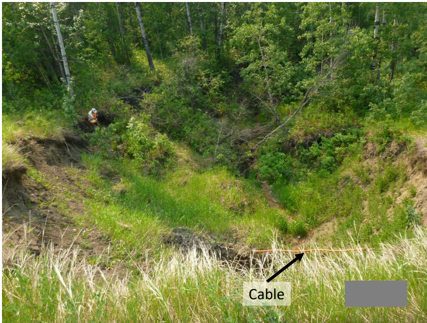
Photo 10 Sinkhole next to inlet of drainage gallery in median backslope of Hwy 43:04. Photo taken June 3, 2025, facing south.
