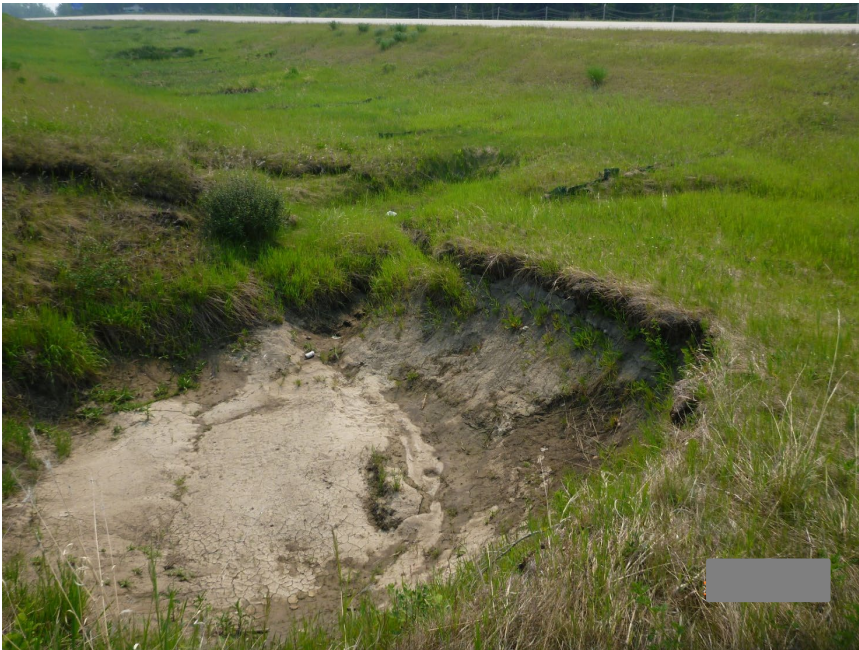
Photo 8 Erosion gully at 0.9-m diameter SWSP culvert outlet on west slope of Hwy 43:04. Note overhang of culvert outlet. Photo taken June 3, 2025, facing southwest.
