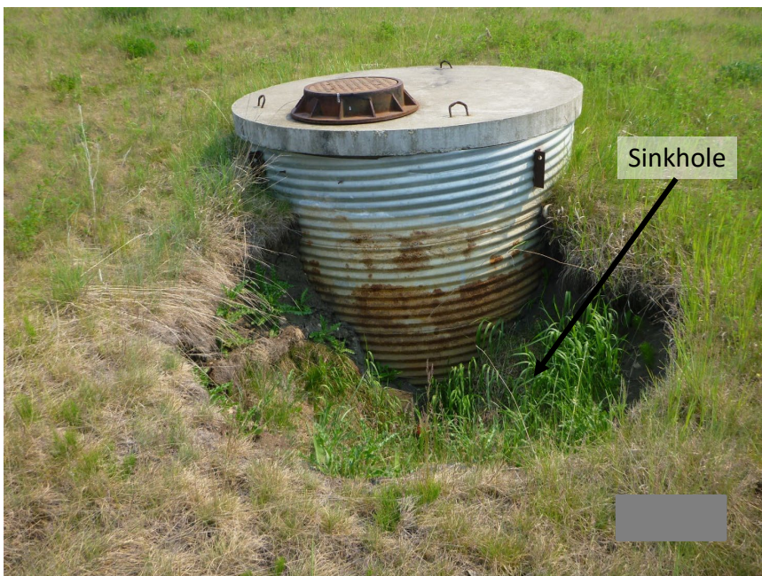
Photo 10 Sinkhole next to inlet of drainage gallery in median backslope of Hwy 43:04. Photo taken June 3, 2025, facing south.
