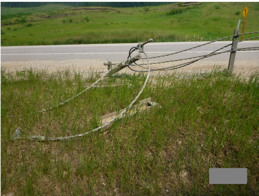
Photo 12 Damaged high-tension cable barrier (HTCB) along west side of southbound lanes of Hwy 43:04. Photo taken June 3, 2025, facing east.
