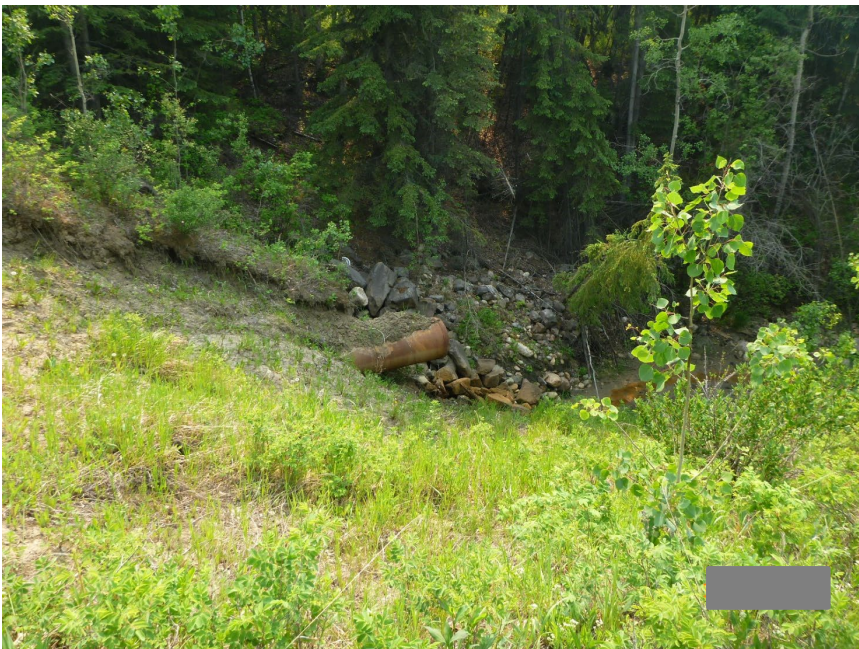
Photo 8 Erosion gully at 0.9-m diameter SWSP culvert outlet on west slope of Hwy 43:04. Note overhang of culvert outlet. Photo taken June 3, 2025, facing southwest.
