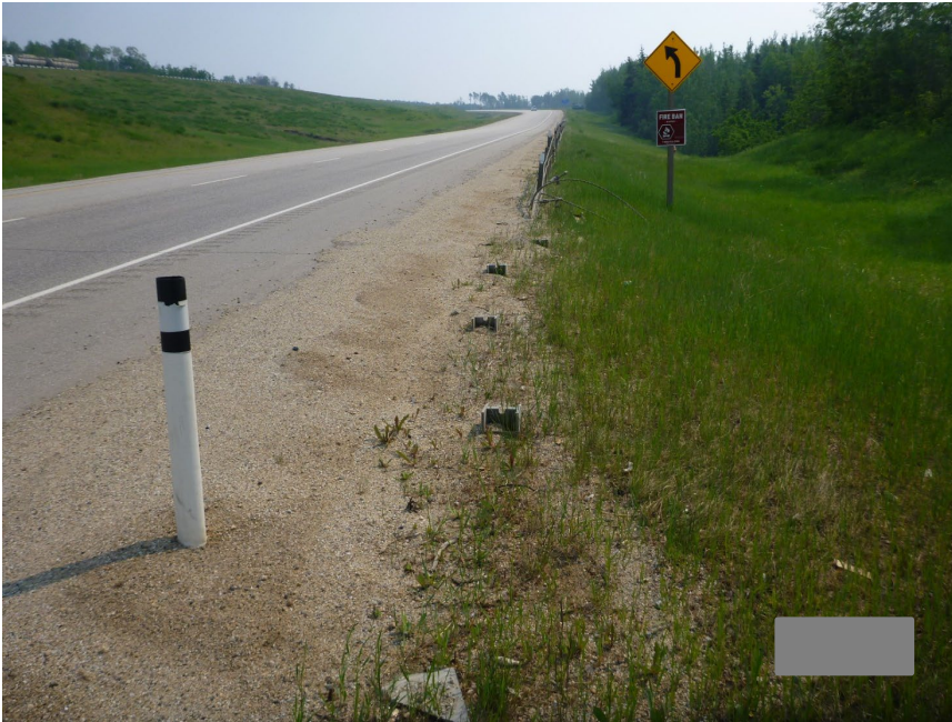
Photo 12 Damaged high-tension cable barrier (HTCB) along west side of southbound lanes of Hwy 43:04. Photo taken June 3, 2025, facing east.
