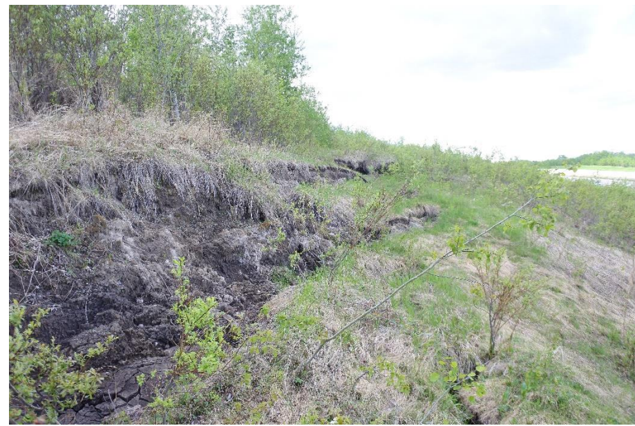
Photo 13. Looking west across the backscarp from the west side of Slide 4. The drop at the backscarp about 1 to 1.5 m in the west half of the slide.
