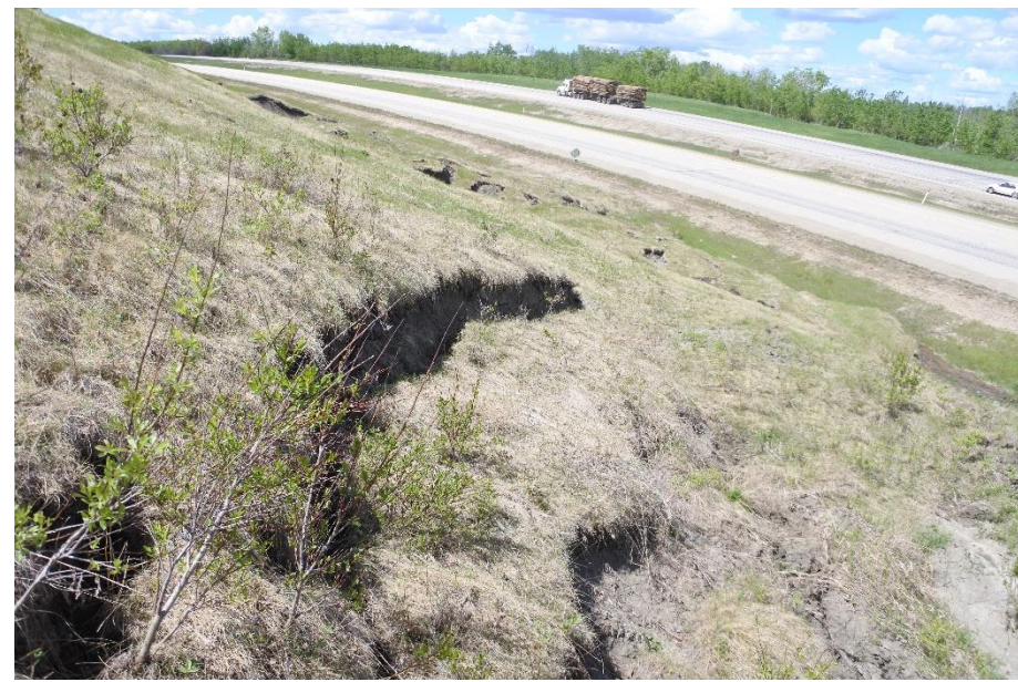
Photo 11. Looking west across the backscarp from the east side of Slide 3. The drop at the backscarp about 2 m in the east half of the slide.
