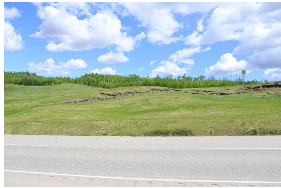
Photo 15. Looking south at east end of Slide 3 which was the least active in 2020.
