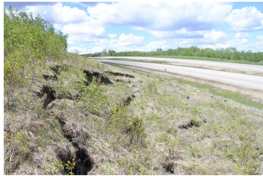
Photo 8. Looking west from the west side of Slide 3. The height of the drop along the backscarp varies from 1 m to 2 m in the western half of Slide 3.
