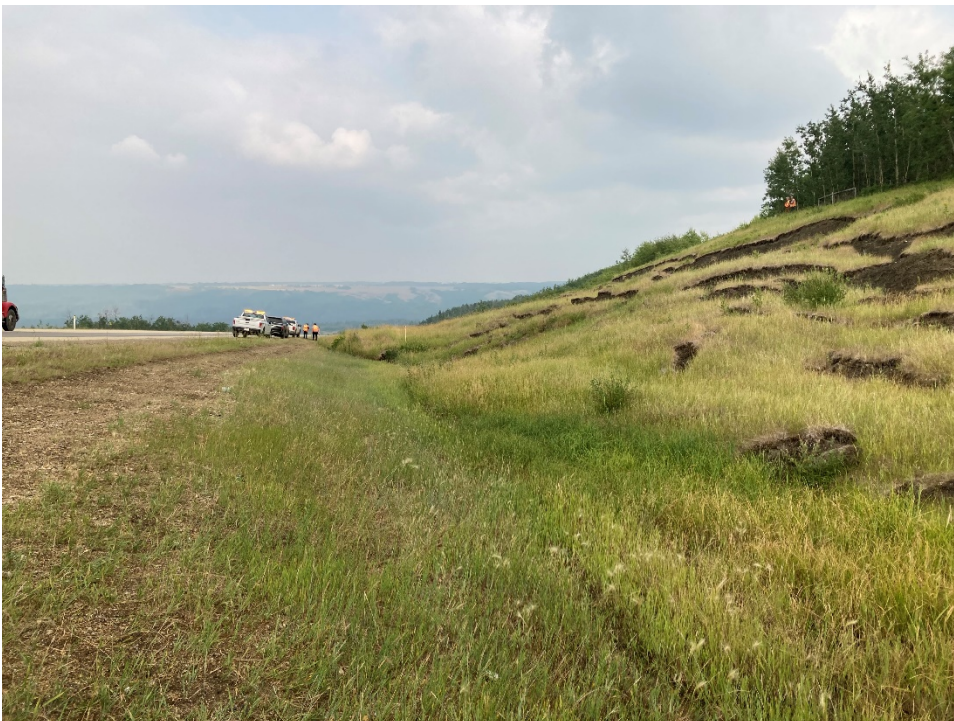
Photo 2 The toe of the slide is blocking the south (eastbound) ditch. Photo taken July 19, 2021 facing east.
