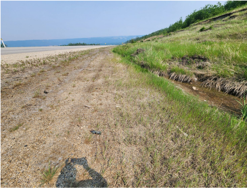
Photo 8 Erosion in ditch at toe of backslope on south side of Hwy 43:04. Photo taken June 3, 2025, facing east.
