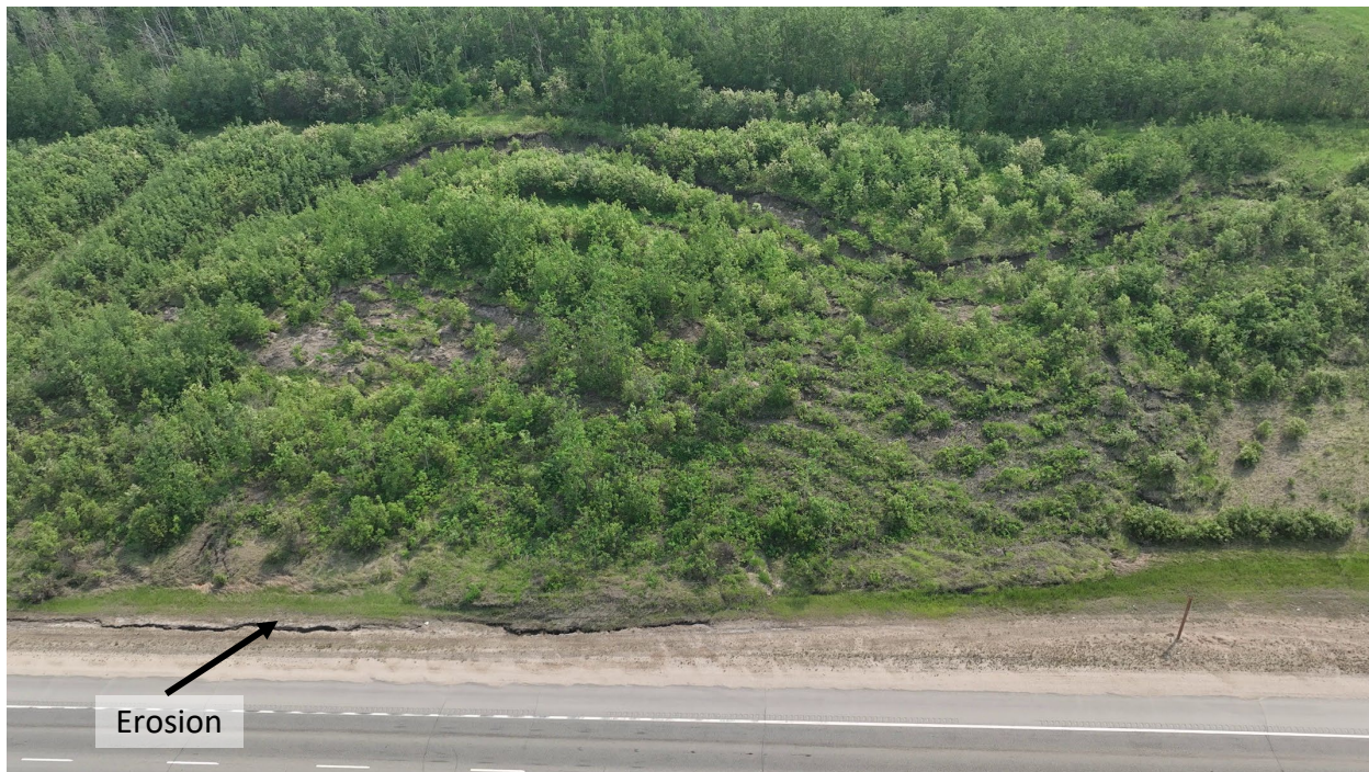
Photo 6 Slope failures along backslope on south side of Hwy 43:04. Note toe rolls in highway ditch. UAV photo taken June 3, 2025, facing south.
