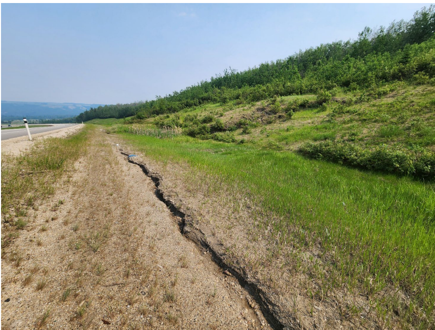
Photo 8 Erosion in ditch at toe of backslope on south side of Hwy 43:04. Photo taken June 3, 2025, facing east.
