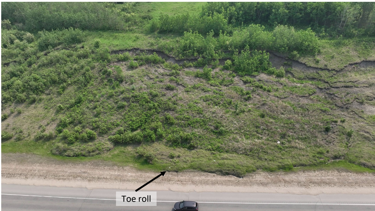
Photo 4 Slope failures along backslope on south side of Hwy 43:04. Note toe rolls in highway ditch. UAV photo taken June 3, 2025, facing south.
