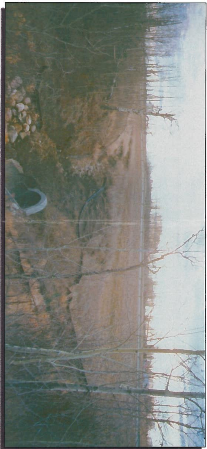
Photo 4 Looking east at east ditch down u/s headslope. -Erosion of outfall ditch.
