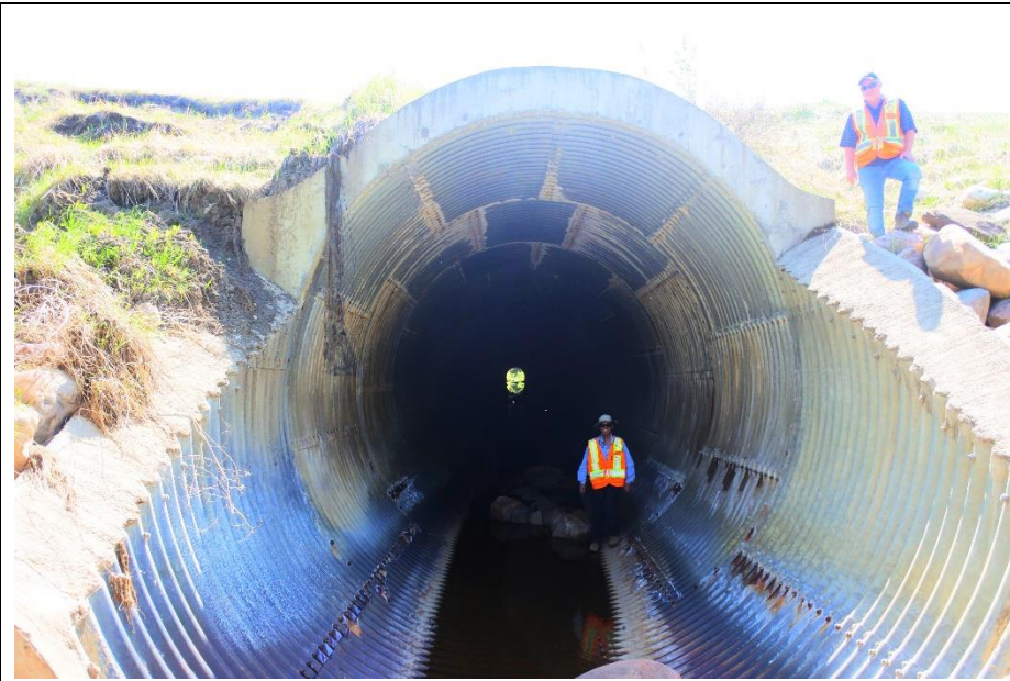
Photo 7. Looking south at culvert inlet.
