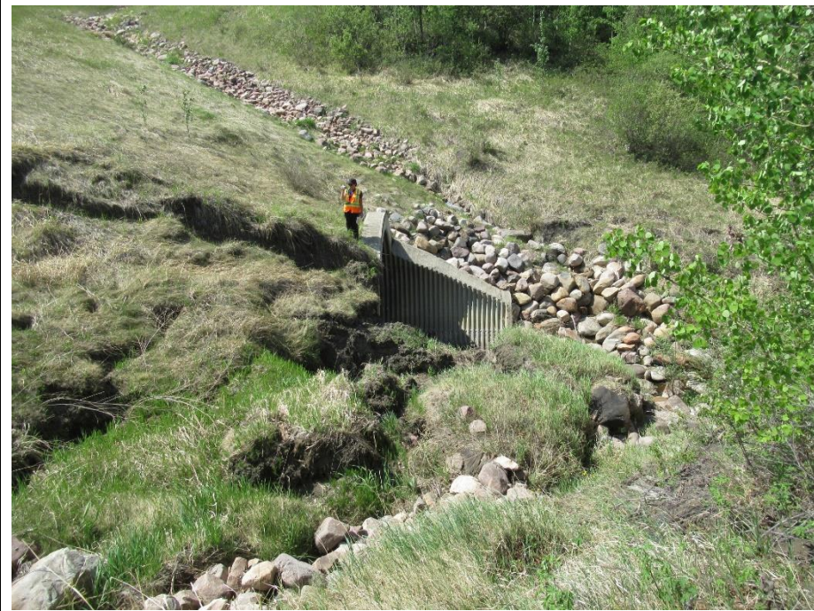
Photo 4. Looking west towards culvert inlet and slide mass.
