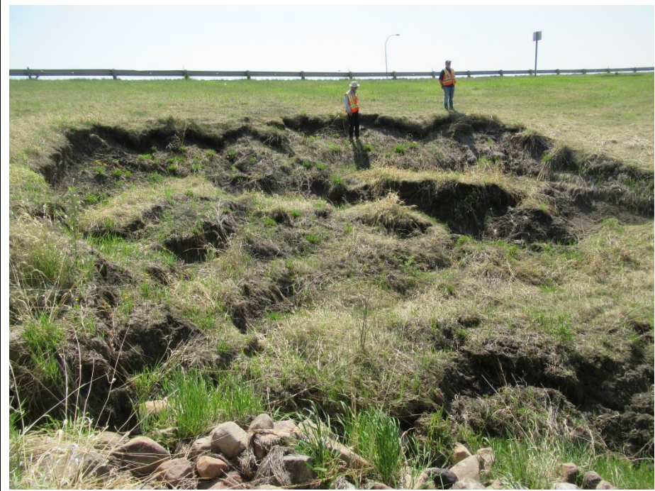
Photo 5. Looking south towards slide and Highway 43.
