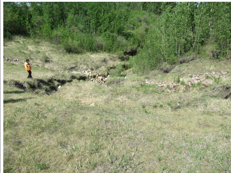
Photo 2. Looking north at slide standing above the backscarp.
