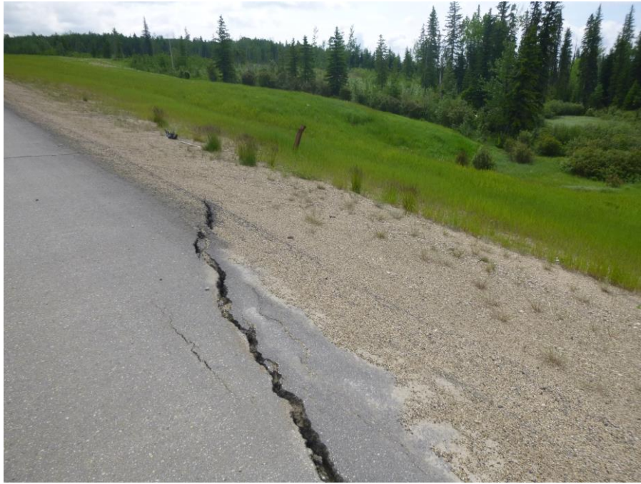
Photo 9 - Looking southeast at the main scarp crack along the south edge of the pavement. Note the subtle scarp extending southeast of the hwy along the top edge of the knob.
