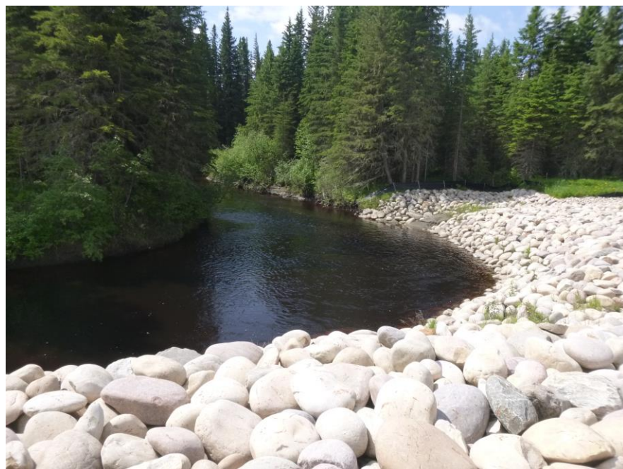
Photo 12 – Looking southwest at the riprap armour. The creek flows adjacent to the front face of the riprap, however no erosion has taken place on the unprotected bank.
