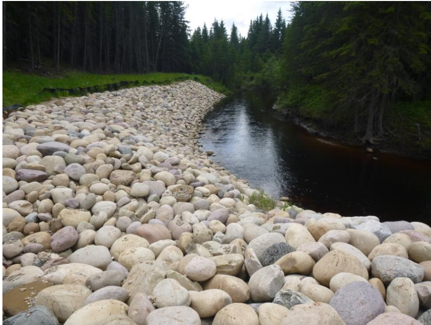
Photo 11 - Looking southeast across the riprap armoured the creek.
