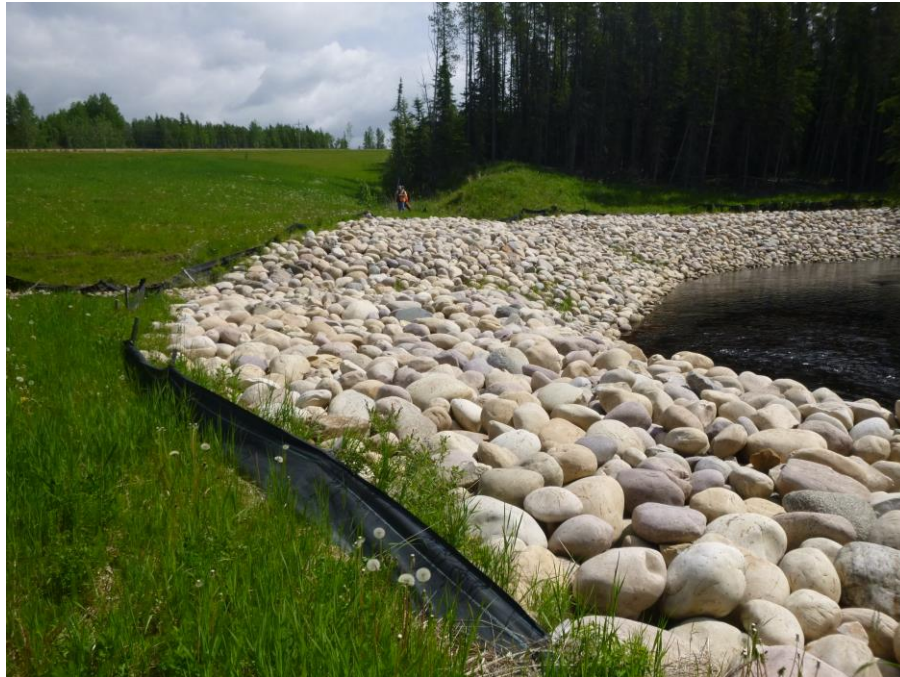
Photo 13 – Looking east across the riprap armour.
