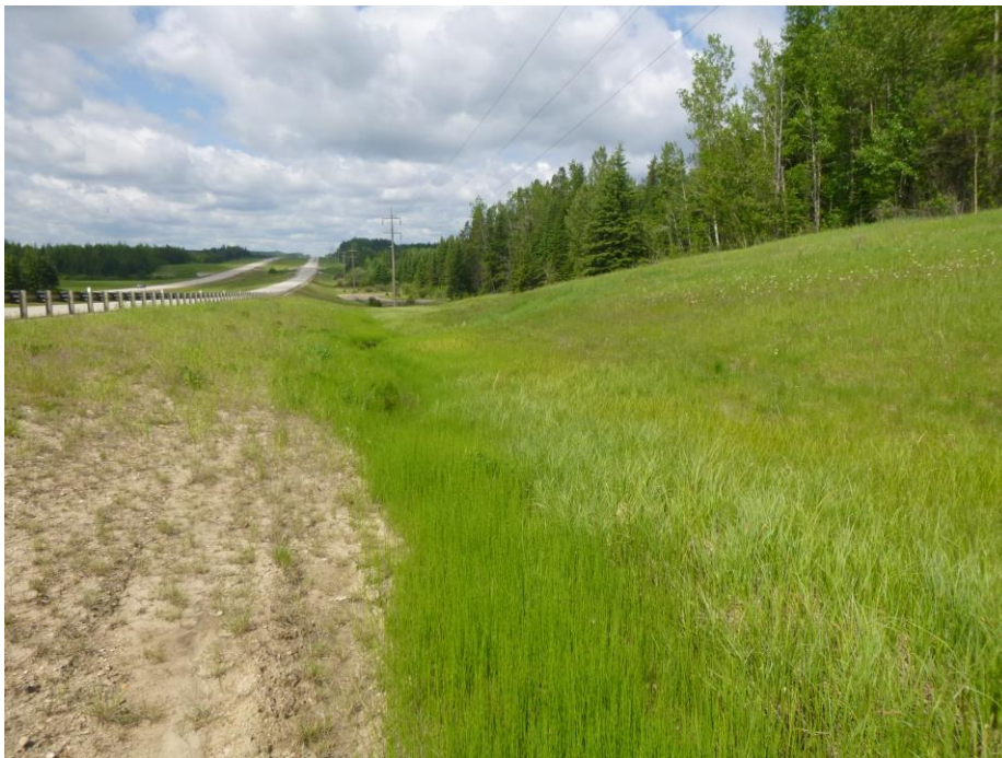
Photo 2 – Looking west along the north ditch at former erosion from flow further east that has grassed in.
