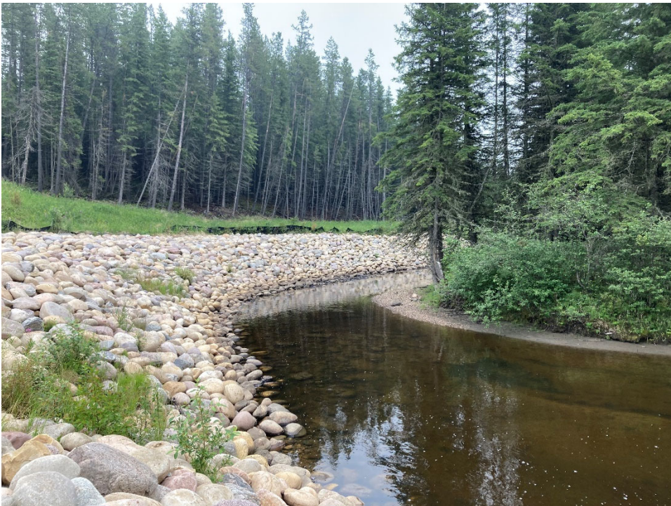
Photo 4 The riprap at the toe of the highway embankment and outside bend of the creek is in good condition. Photo taken July 19, 2021, facing southeast.
