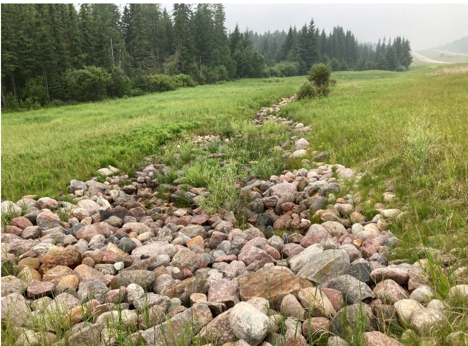
Photo 2 The riprap lined channel at the outlet of the drain pipe underlying the eastbound lanes of Hwy 43. Photo taken July 19, 2021, facing west.
