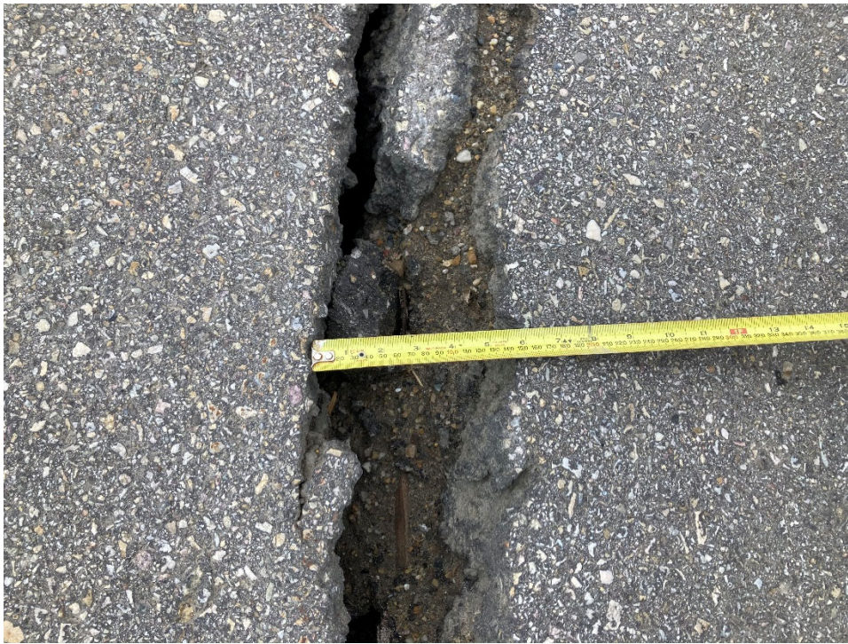
Photo 8 A delineator post was inserted into the asphalt crack at the edge of the highway before the 2021 inspection. Photo taken July 19, 2021, facing north.
