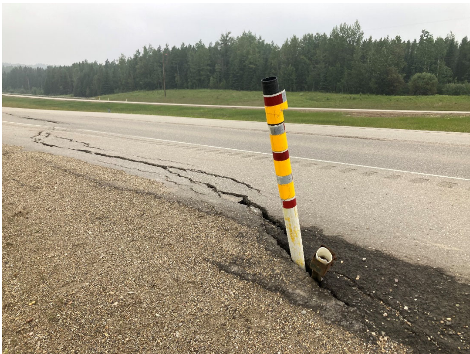
Photo 8 A delineator post was inserted into the asphalt crack at the edge of the highway before the 2021 inspection. Photo taken July 19, 2021, facing north.
