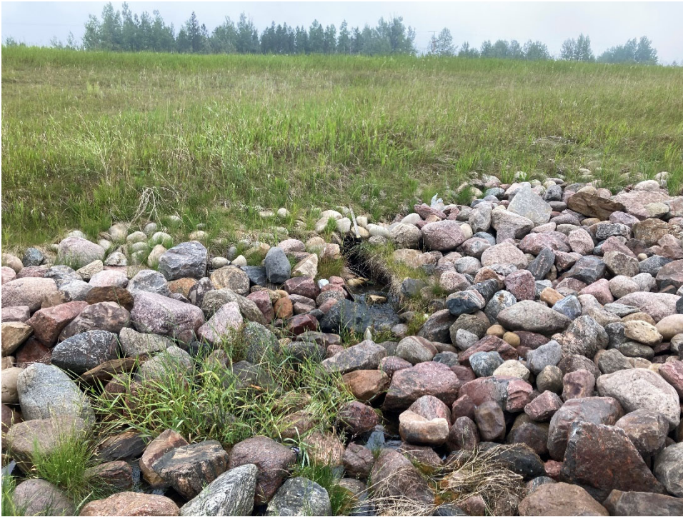
Photo 4 The riprap at the toe of the highway embankment and outside bend of the creek is in good condition. Photo taken July 19, 2021, facing southeast.
