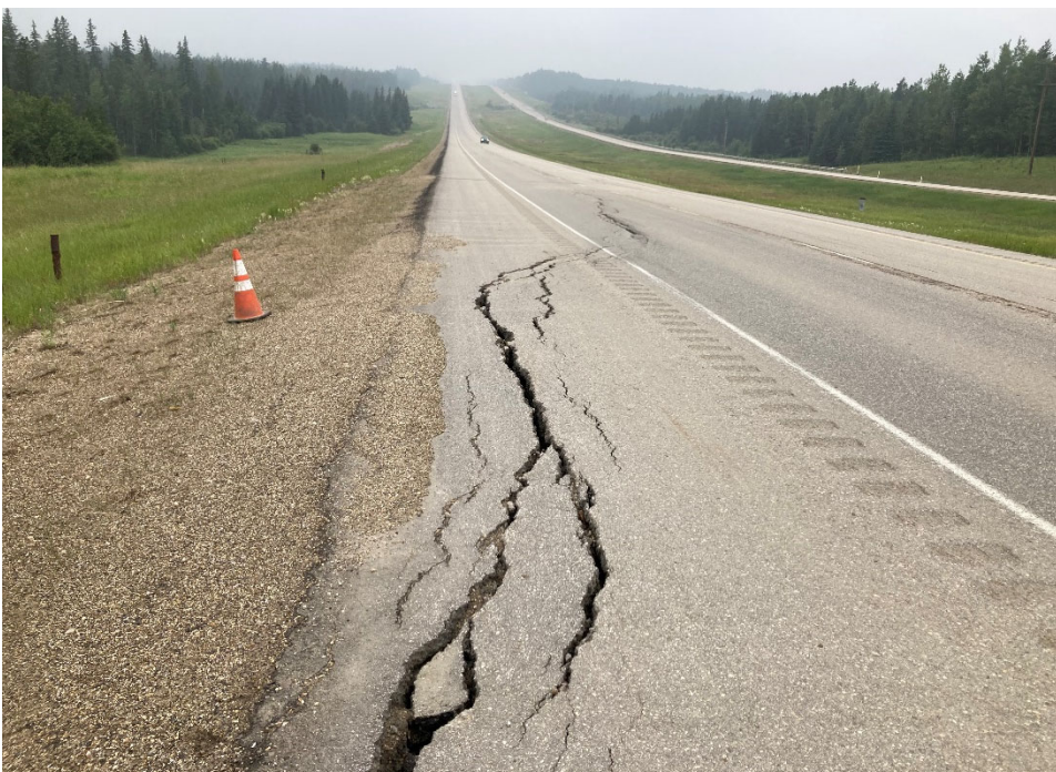
Photo 6 Asphalt cracking in the eastbound travel lane extends from the edge of the asphalt to the centreline. The cracking has worsened since the 2020 inspection. Photo taken July 19, 2021, facing west.
