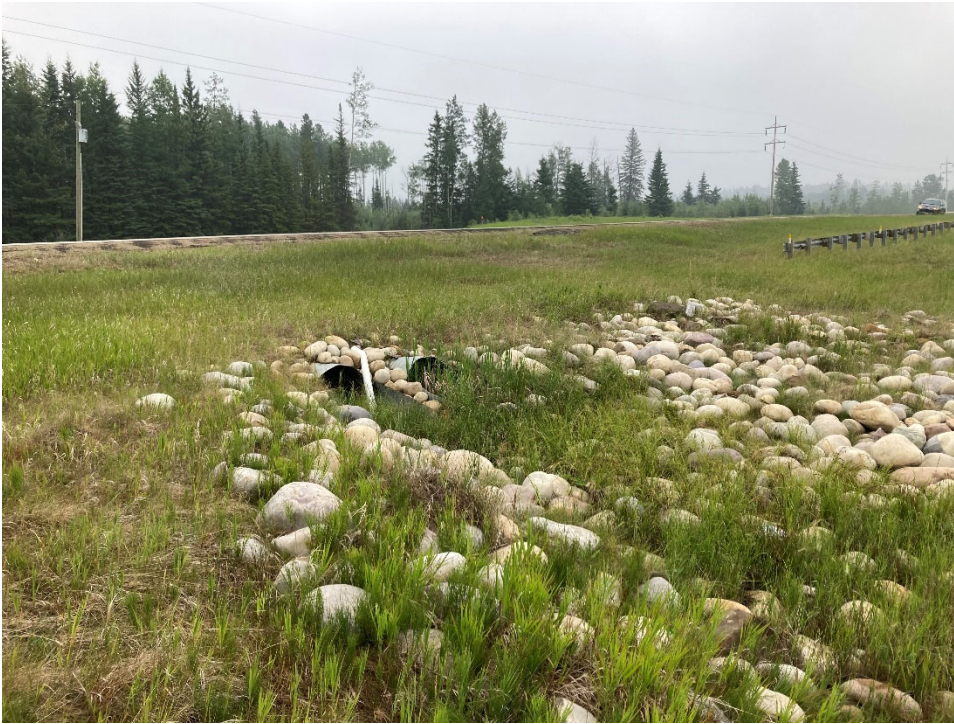
Photo 2 The riprap lined channel at the outlet of the drain pipe underlying the eastbound lanes of Hwy 43. Photo taken July 19, 2021, facing west.
