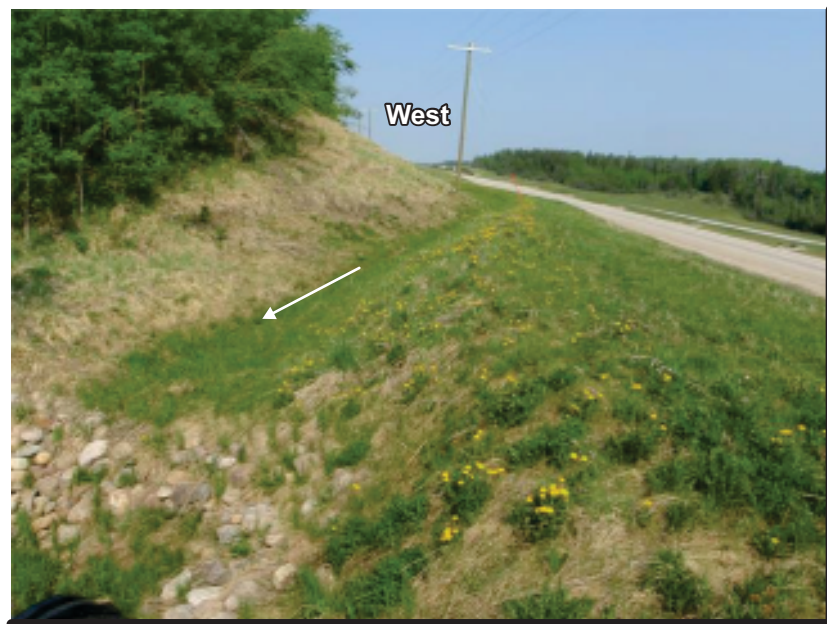
Photo 2b Catchwater Ditch inflow sections (east end and west end)
