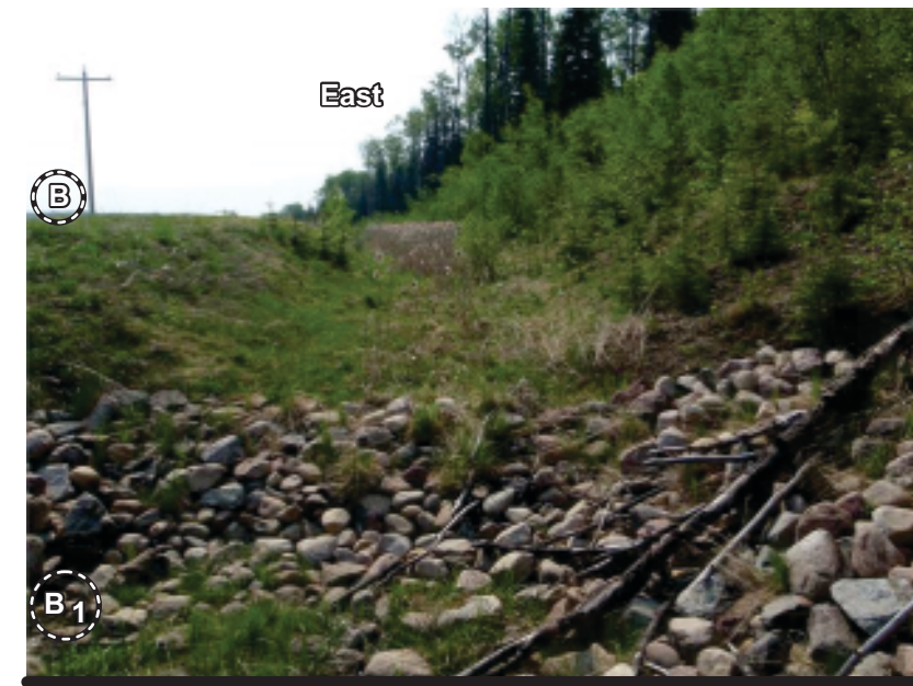
Photo 2a Catchwater Ditch inflow sections (east end and west end)
