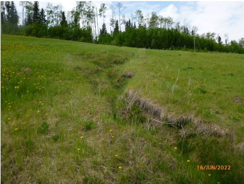
Photo 6 Material slumping, settling, and eroding above “Big-O” pipe on backslope along west side of Hwy 43:12. Photo taken June 16, 2022, facing west.
