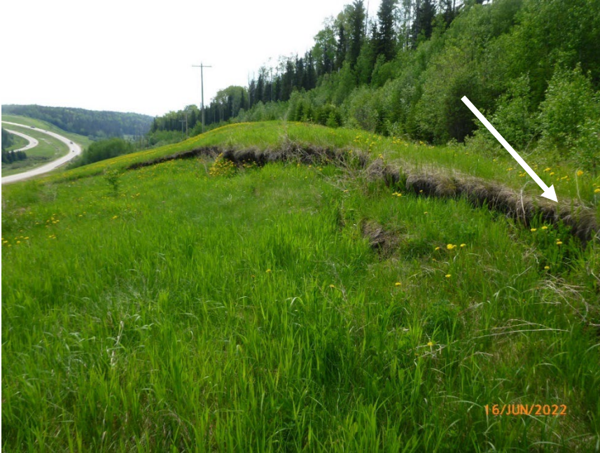
Photo 6 Material slumping, settling, and eroding above “Big-O” pipe on backslope along west side of Hwy 43:12. Photo taken June 16, 2022, facing west.
