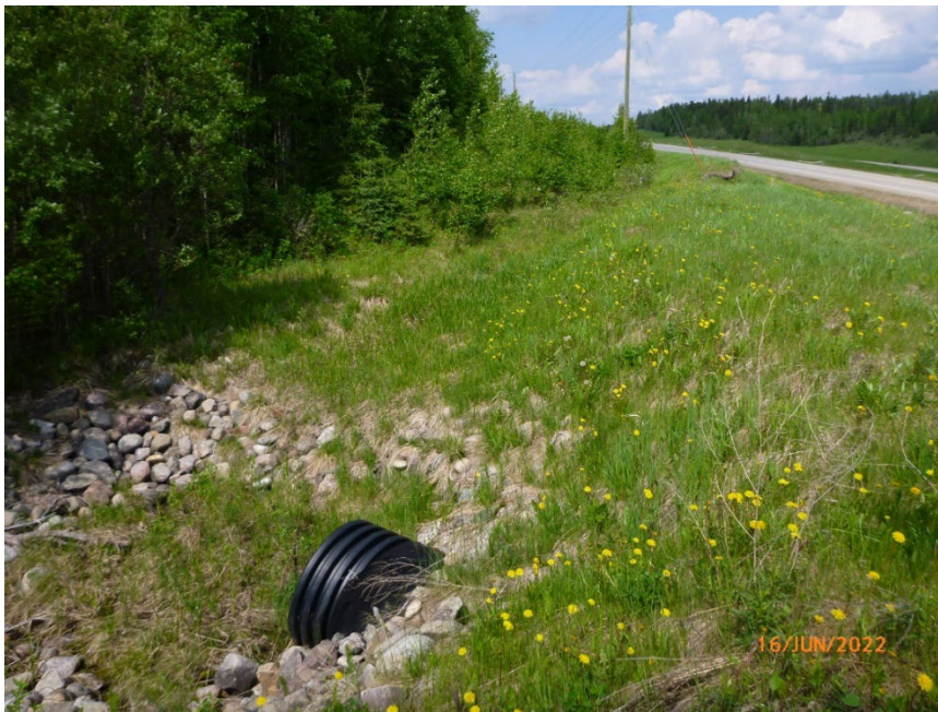
Photo 4 Inlet of “Big-O” pipe at crest of backslope at WP230. Photo taken June 16, 2022, facing northwest.
