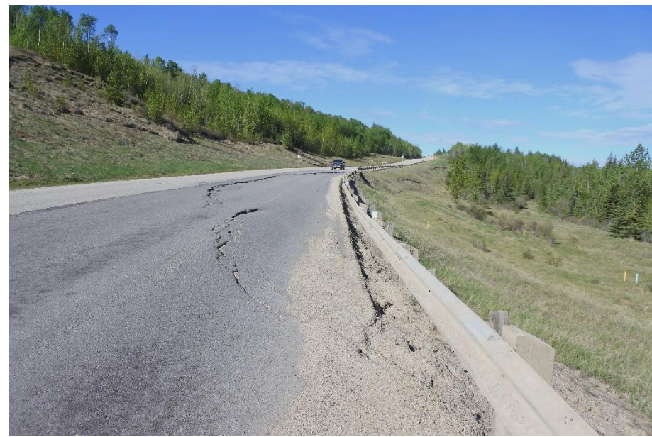
Photo 15. Looking west at the ACP patch in outer WBL at Mid- Valley/" Old Major" Landslide (Site 1).
