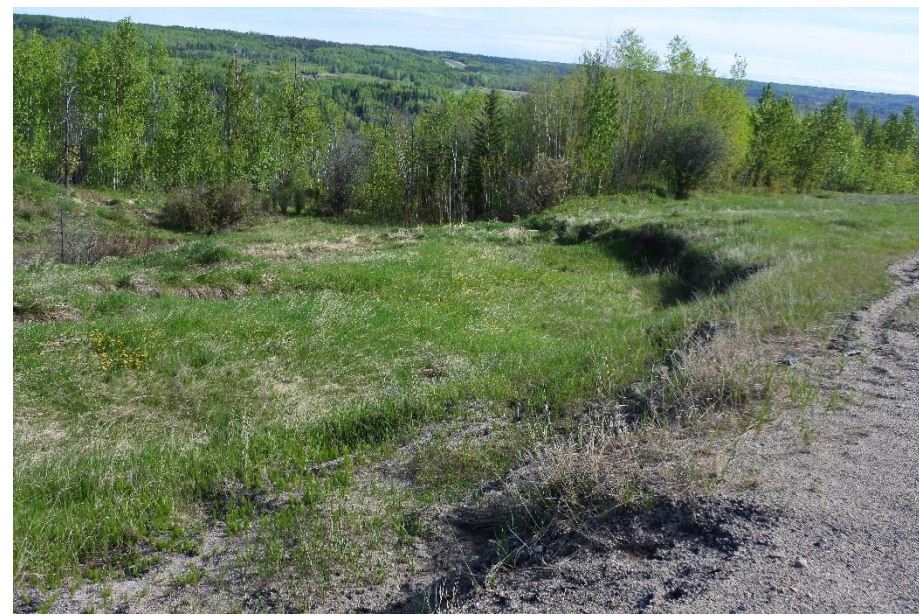
Photo 21. Looking northeast from the shoulder of the WBL at the scarp extending into the brush at the Valley Top Landslide (Site 3).
