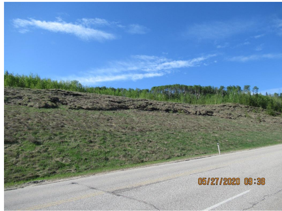
Photo 14. Looking southwest from the WBL shoulder at the slide in the backslope in the eastern portion off the Mid-Valley/" Old Major" Landslide (Site 1).
