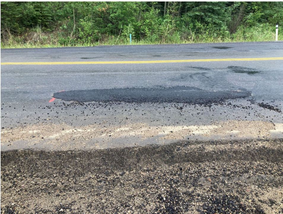
Photo 4 A recent patch at WP 0087 completed in the north (westbound) lane in spring 2021 after cracking and a sinkhole (void under pavement) was observed by the Maintenance Contract Inspector (MCI). Photo taken July 20, 2021 facing south.
