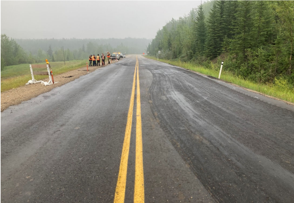
Photo 2 Asphalt cracking observed near the east extent of the lower slide, running diagonally across the highway. Photo taken July 20, 2021 facing east.
