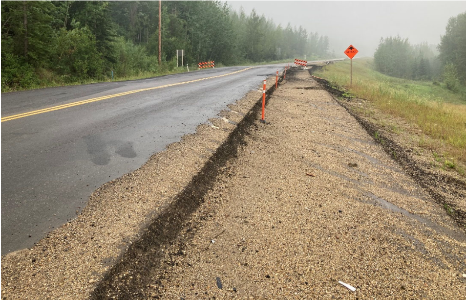
Photo 4 A recent patch at WP 0087 completed in the north (westbound) lane in spring 2021 after cracking and a sinkhole (void under pavement) was observed by the Maintenance Contract Inspector (MCI). Photo taken July 20, 2021 facing south.
