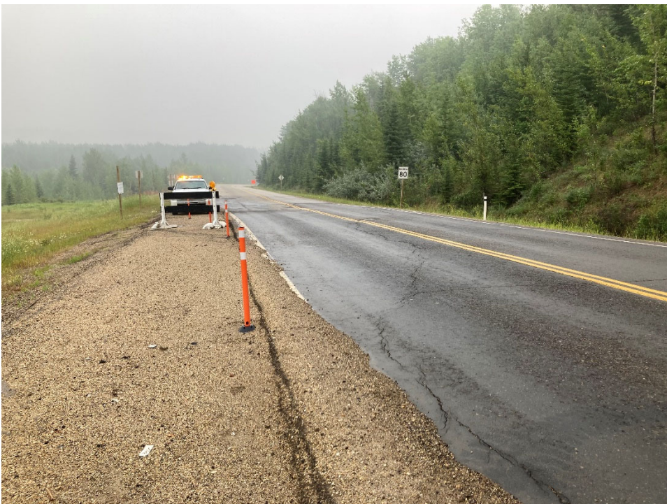
Photo 2 Asphalt cracking observed near the east extent of the lower slide, running diagonally across the highway. Photo taken July 20, 2021 facing east.
