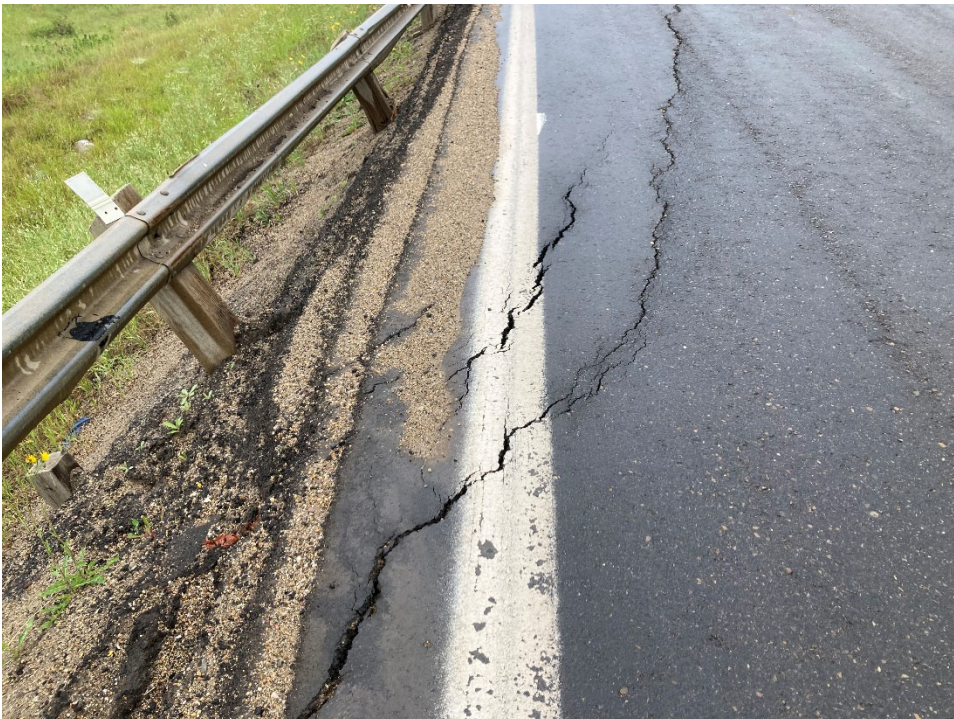
Photo 8 A close-up photo of the asphalt cracking observed near the west extent of the asphalt patch (shown in Photo 8). Photo taken July 20, 2021 facing east.
