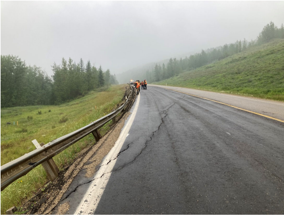
Photo 8 A close-up photo of the asphalt cracking observed near the west extent of the asphalt patch (shown in Photo 8). Photo taken July 20, 2021 facing east.
