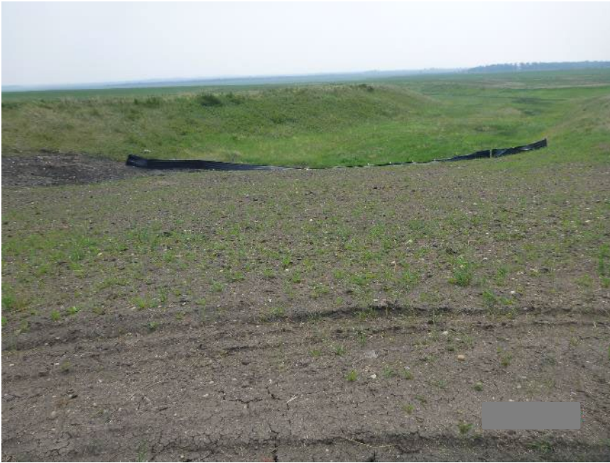
Photo 6 Slope of toe berm constructed in 2024 on south side of Hwy 674:02. Note poor vegetation cover. Photo taken June 3, 2025, facing northeast.
