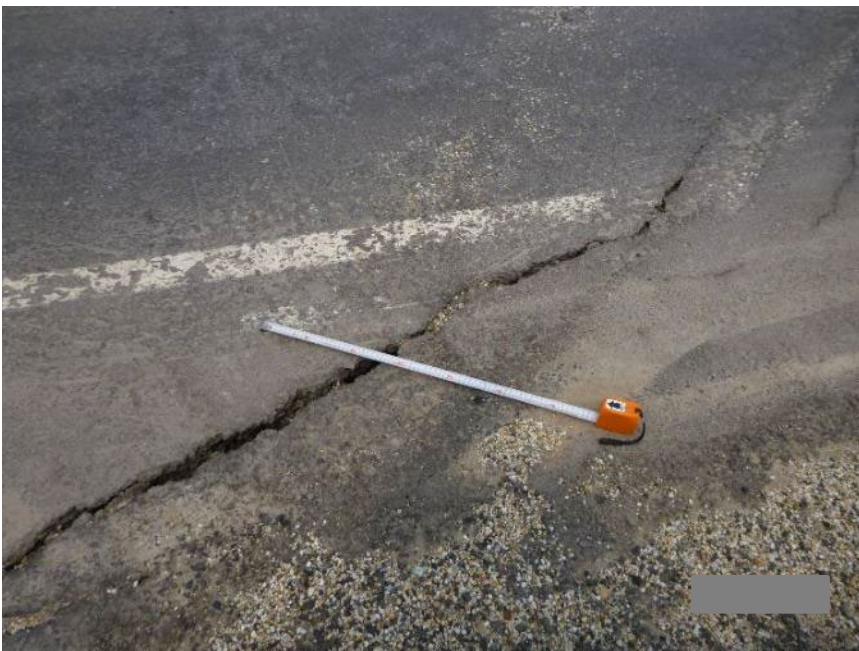
Photo 4 Cracking in eastbound lane of Hwy 674:02 through pavement patch placed in October 2024. Photo taken June 3, 2025.
