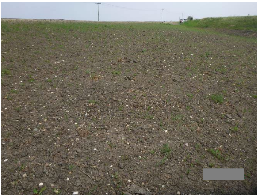
Photo 6 Slope of toe berm constructed in 2024 on south side of Hwy 674:02. Note poor vegetation cover. Photo taken June 3, 2025, facing northeast.
