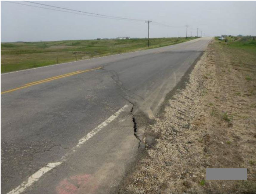
Photo 4 Cracking in eastbound lane of Hwy 674:02 through pavement patch placed in October 2024. Photo taken June 3, 2025.
