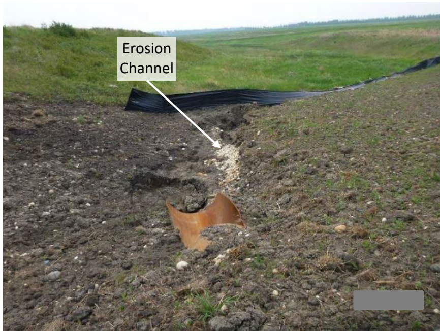
Photo 8 Erosion channel downstream of culvert outlet extended in 2024. Note silt fence being undermined by erosion. Photo taken June 3, 2025, facing southwest.
