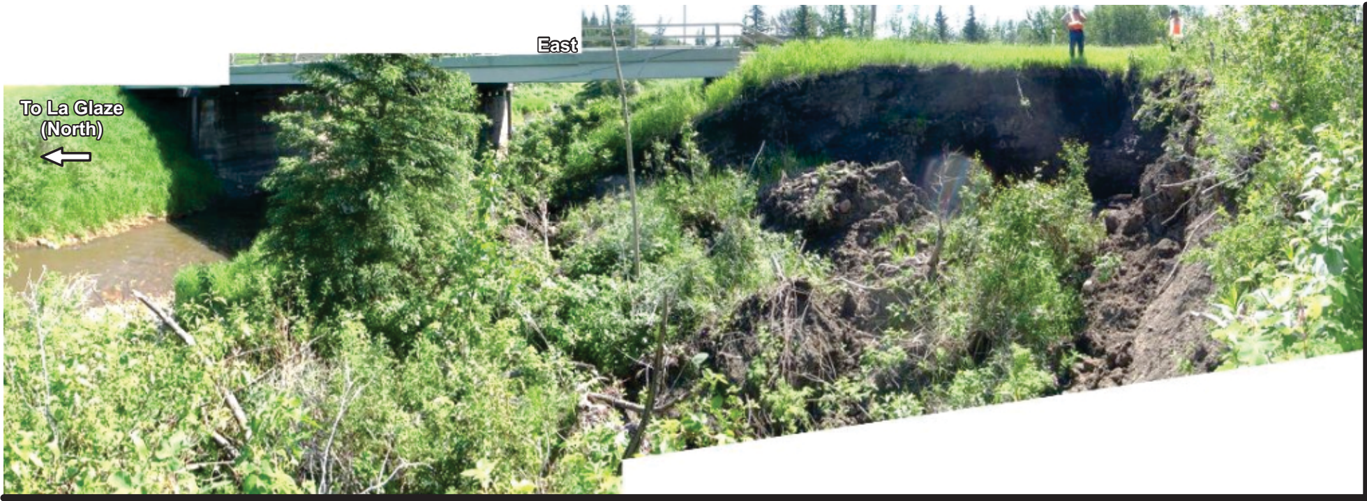
Photo IV Looking east - another view of slide • Width of slide at about 30-35m • Height of slide (valley slope) at about 7-10m
