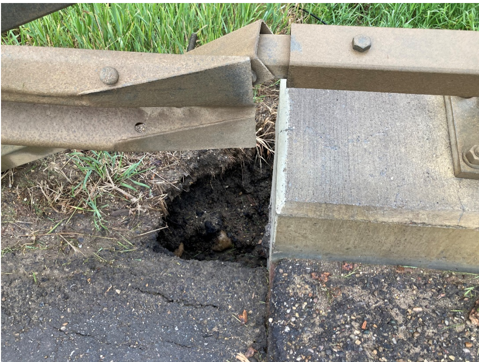
Photo 10 Erosion at the southwest corner (west side of the south abutment) of the bridge crossing Colquhoun Creek. Photo taken July 20, 2021 facing west,
