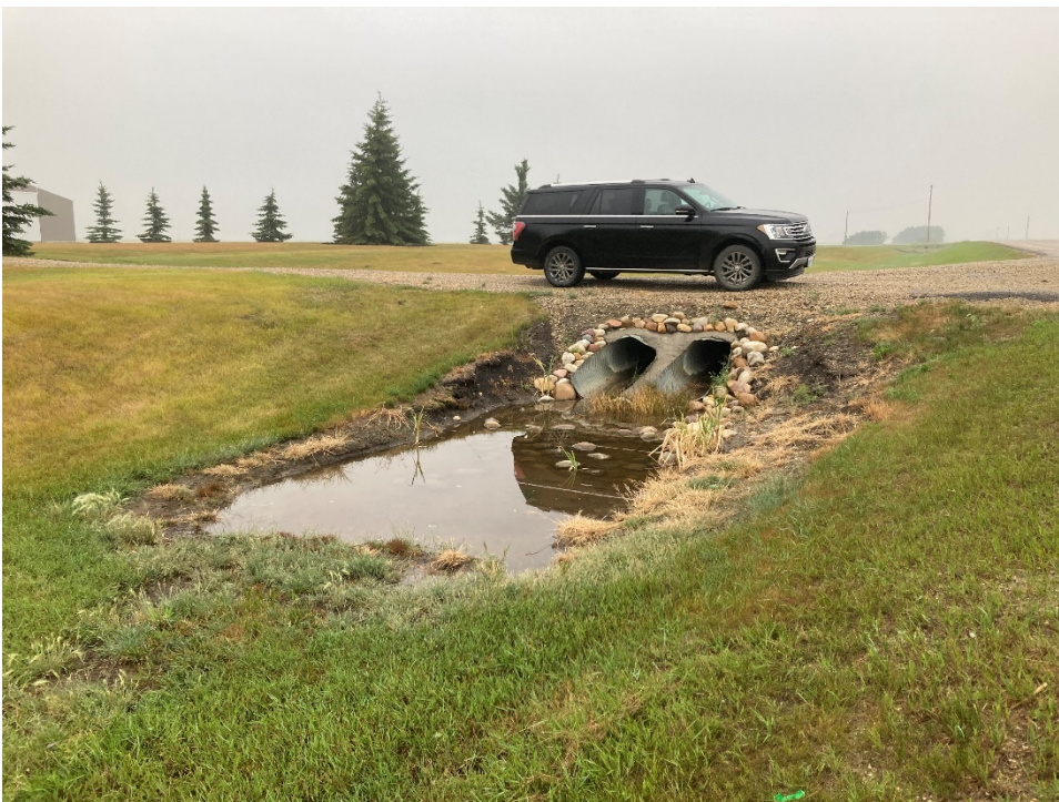
Photo 2 Outlet of the twin 800 mm diameter CSP culverts. Water has ponded in the riprap apron. Photo taken July 20, 2021 facing north.
