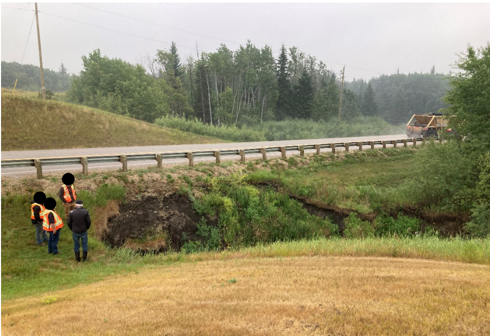
Photo 6 The erosion gully is retrogressing towards the west (southbound) lane and is less than 2 m from the edge of pavement. Photo taken July 20, 2021 facing southeast.
