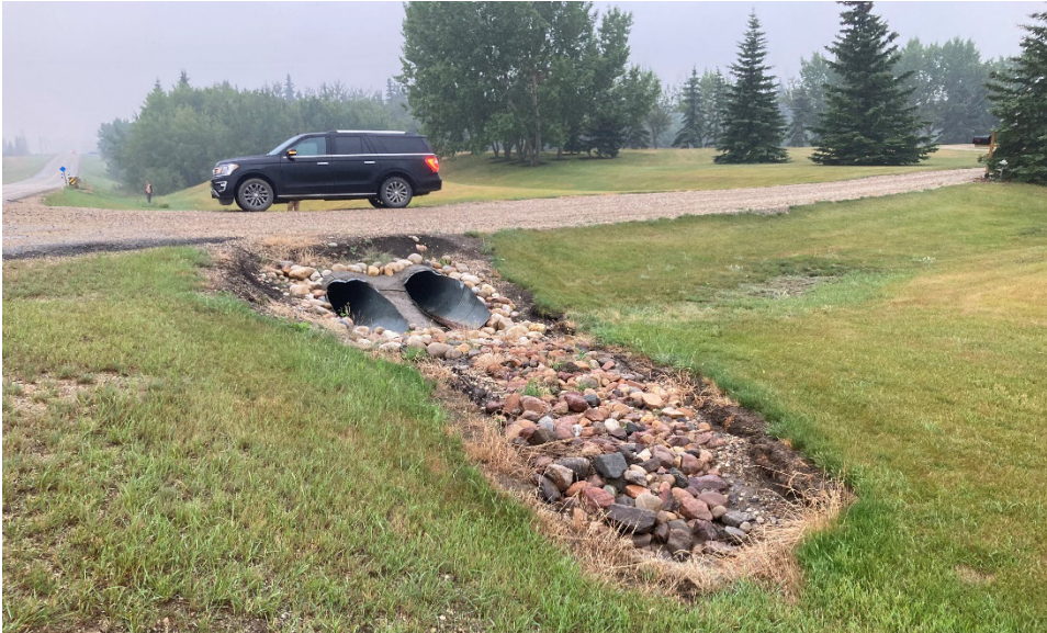
Photo 2 Outlet of the twin 800 mm diameter CSP culverts. Water has ponded in the riprap apron. Photo taken July 20, 2021 facing north.
