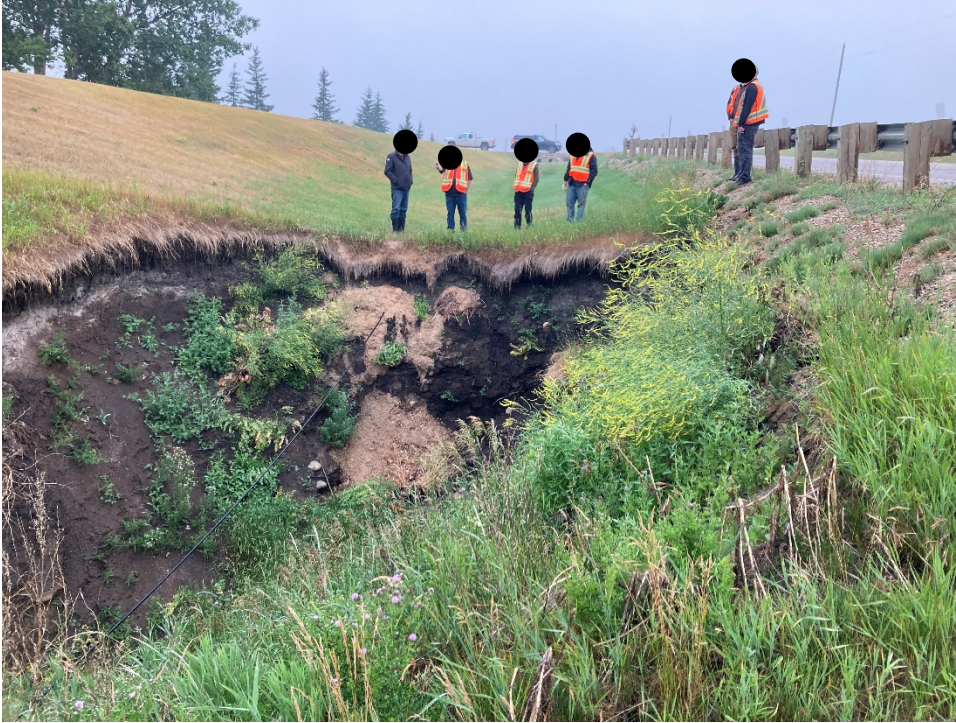
Photo 6 The erosion gully is retrogressing towards the west (southbound) lane and is less than 2 m from the edge of pavement. Photo taken July 20, 2021 facing southeast.
