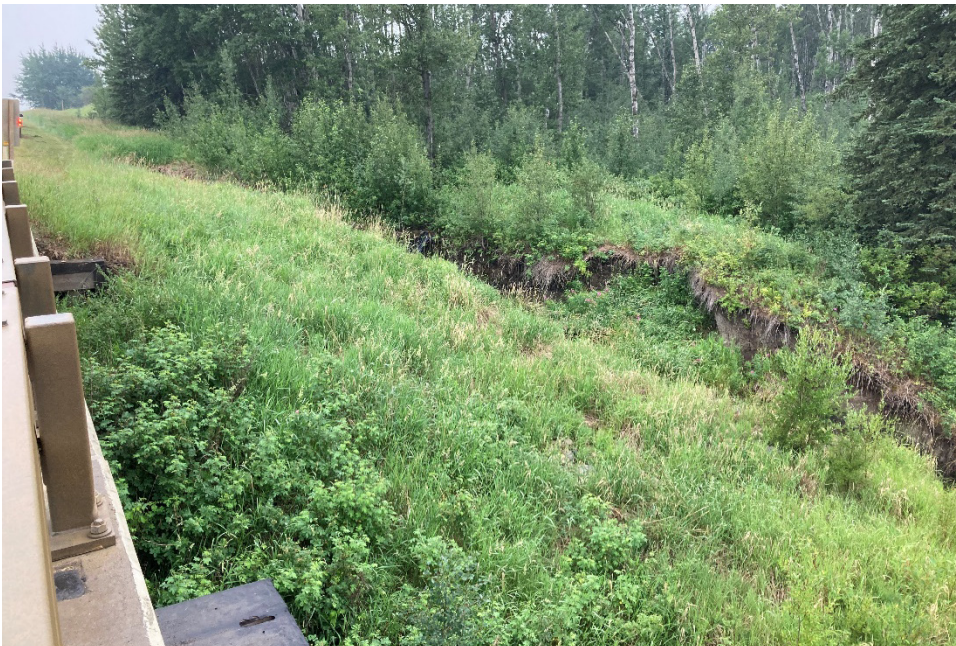
Photo 8 Erosion gully viewed from the south abutment of the bridge crossing Colquhoun Creek. Photo taken July 20, 2021 facing southwest.
