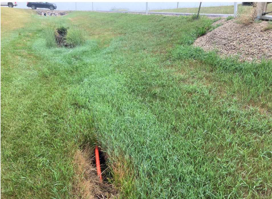
Photo 4 Exposed utility line in the west (southbound) ditch. The utility line is still exposed from hydro-vacing. Photo taken July 20, 2021 facing north.
