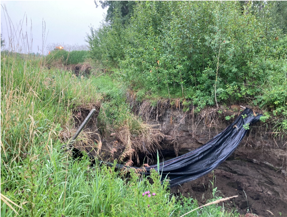
Photo 10 Erosion at the southwest corner (west side of the south abutment) of the bridge crossing Colquhoun Creek. Photo taken July 20, 2021 facing west,
