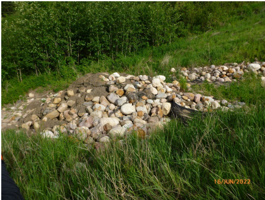
Photo 6 Displaced riprap deposited in pile near bottom of ditch channel. Photo taken June 16, 2022, facing northwest.
