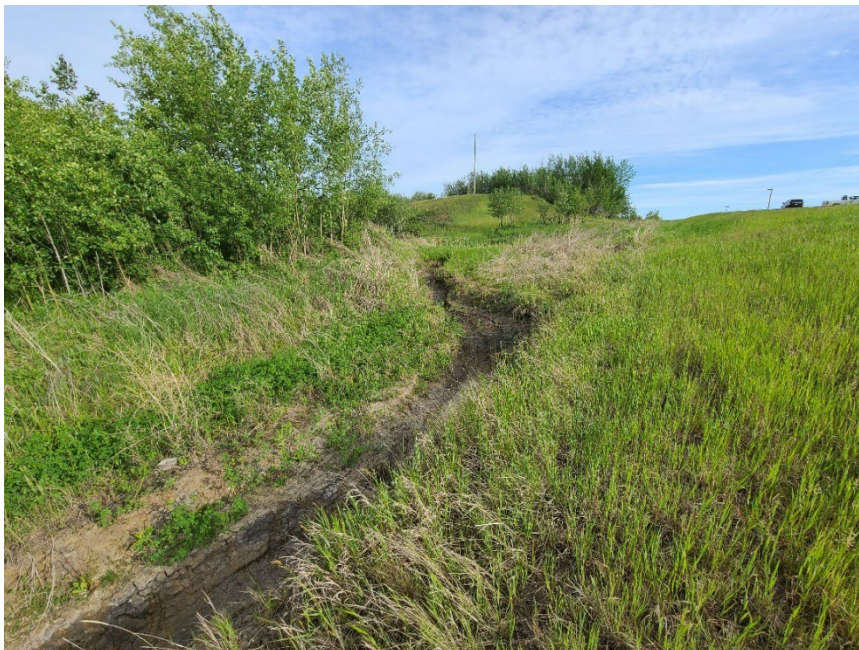
Photo 2 Channel approximately 0.3 m to 0.5 m deep, 1.0 m wide eroded into west ditch of Hwy 733:02. Photo taken June 16, 2022, facing northwest.
