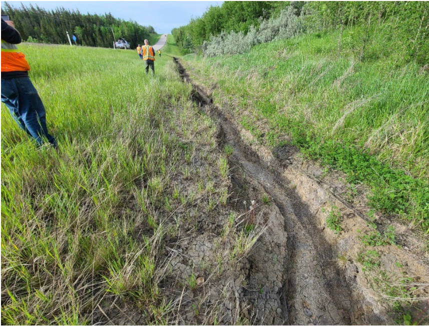
Photo 4 Almost all riprap from previously riprap-lined portion of ditch channel displaced. Note underlying geotechnical is damaged and undermined. Photo taken June 16, 2022, facing northeast looking up northwest embankment abutment.
