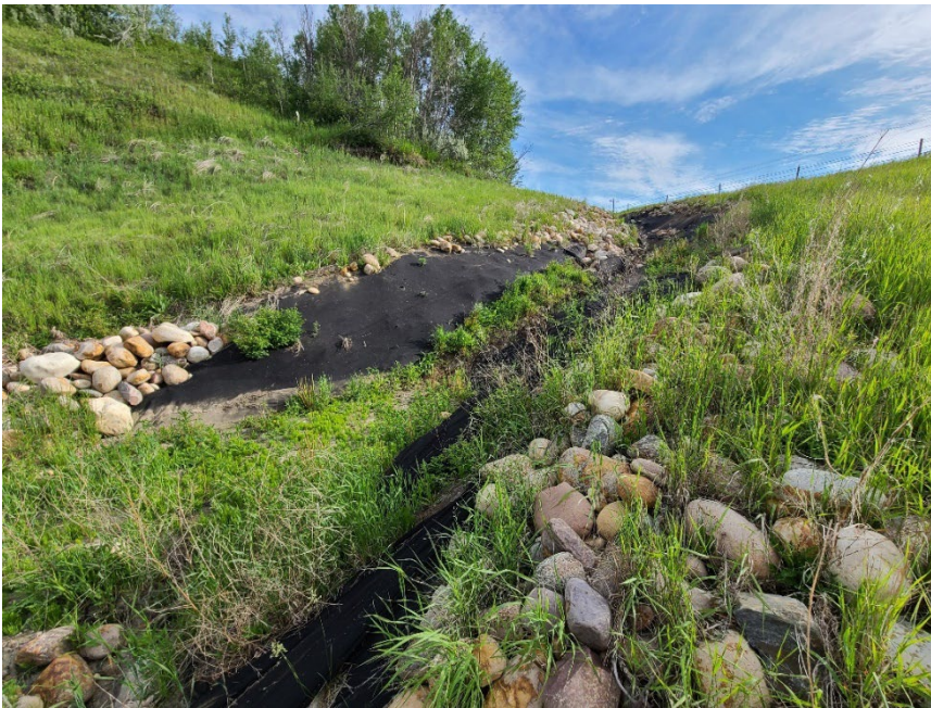
Photo 4 Almost all riprap from previously riprap-lined portion of ditch channel displaced. Note underlying geotechnical is damaged and undermined. Photo taken June 16, 2022, facing northeast looking up northwest embankment abutment.
