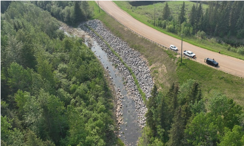
Photo 7 Repaired riverbank erosion on southeast side of Hwy 736:02. Note row of live staking in riprap. Photo taken June 3, 2025, facing southwest.
