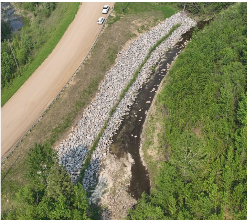
Photo 5 Repaired riverbank erosion on southeast side of Hwy 736:02. Note row of live staking in riprap. UAV photo taken June 3, 2025, facing northeast.
