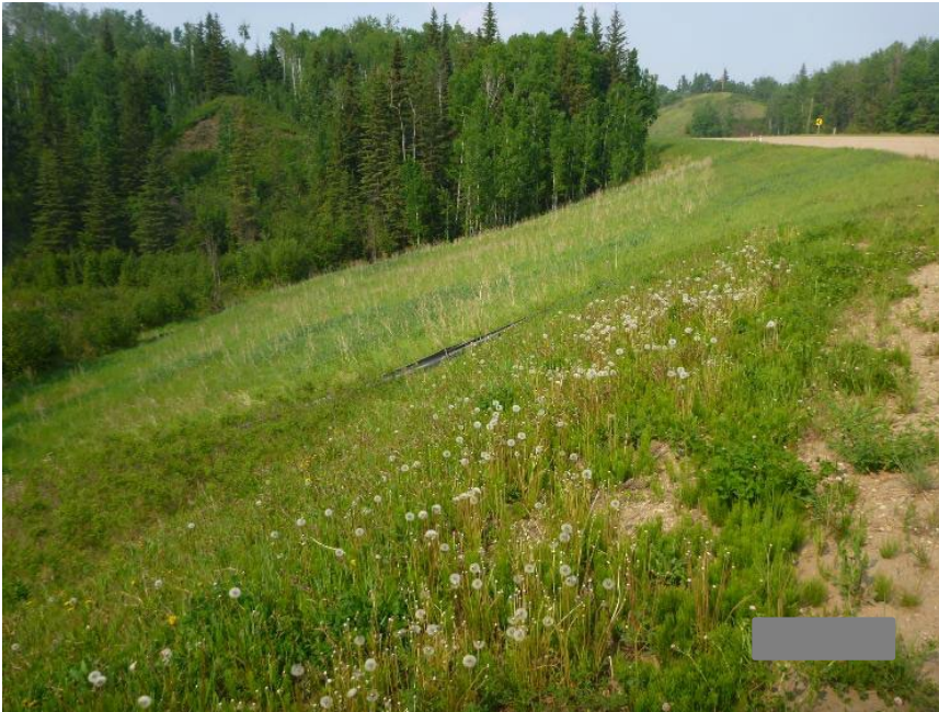
Photo 5 Repaired riverbank erosion on southeast side of Hwy 736:02. Note row of live staking in riprap. UAV photo taken June 3, 2025, facing northeast.
