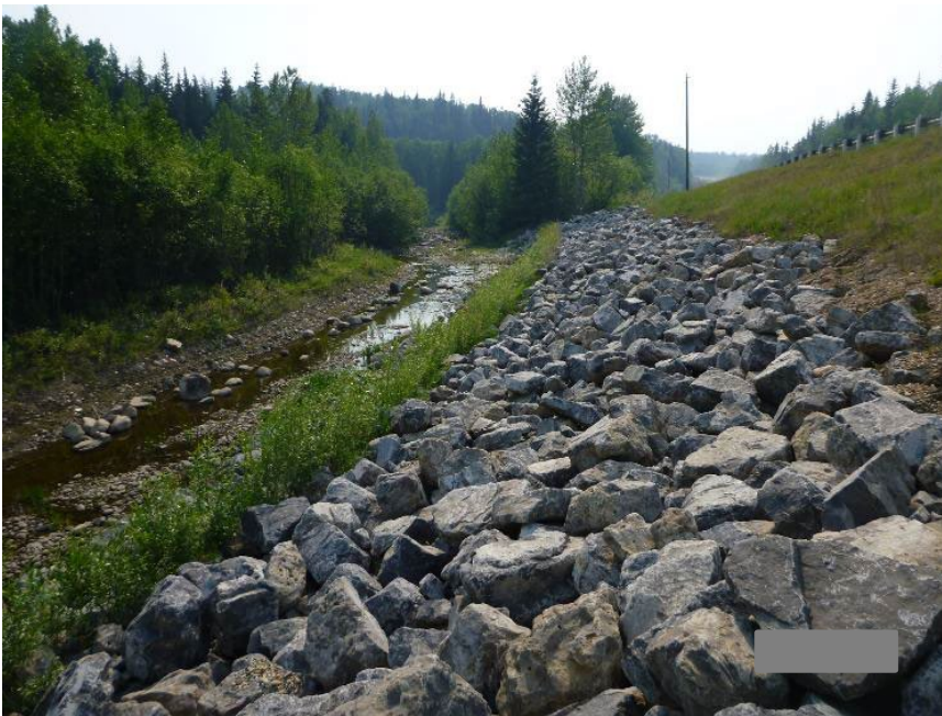
Photo 7 Repaired riverbank erosion on southeast side of Hwy 736:02. Note row of live staking in riprap. Photo taken June 3, 2025, facing southwest.
