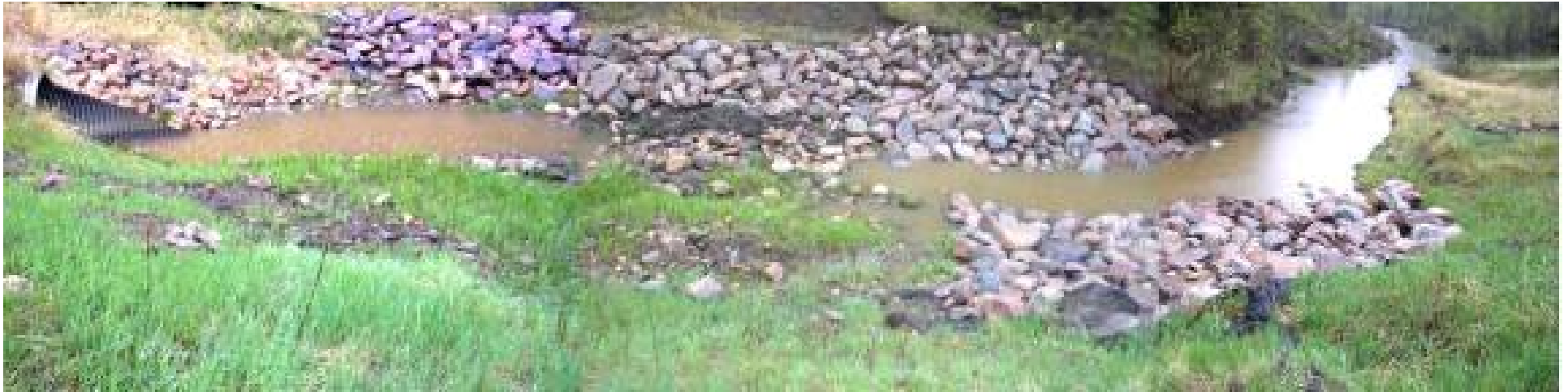
Photo 3 - Panoramic view of the culvert outlet and the Class 2 armour, May 25, 2006.
