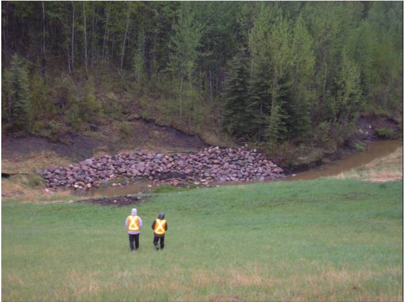
Photo 2 - Southeast view of the additional Class2 riprap at culvert outlet, May 25, 2006.
