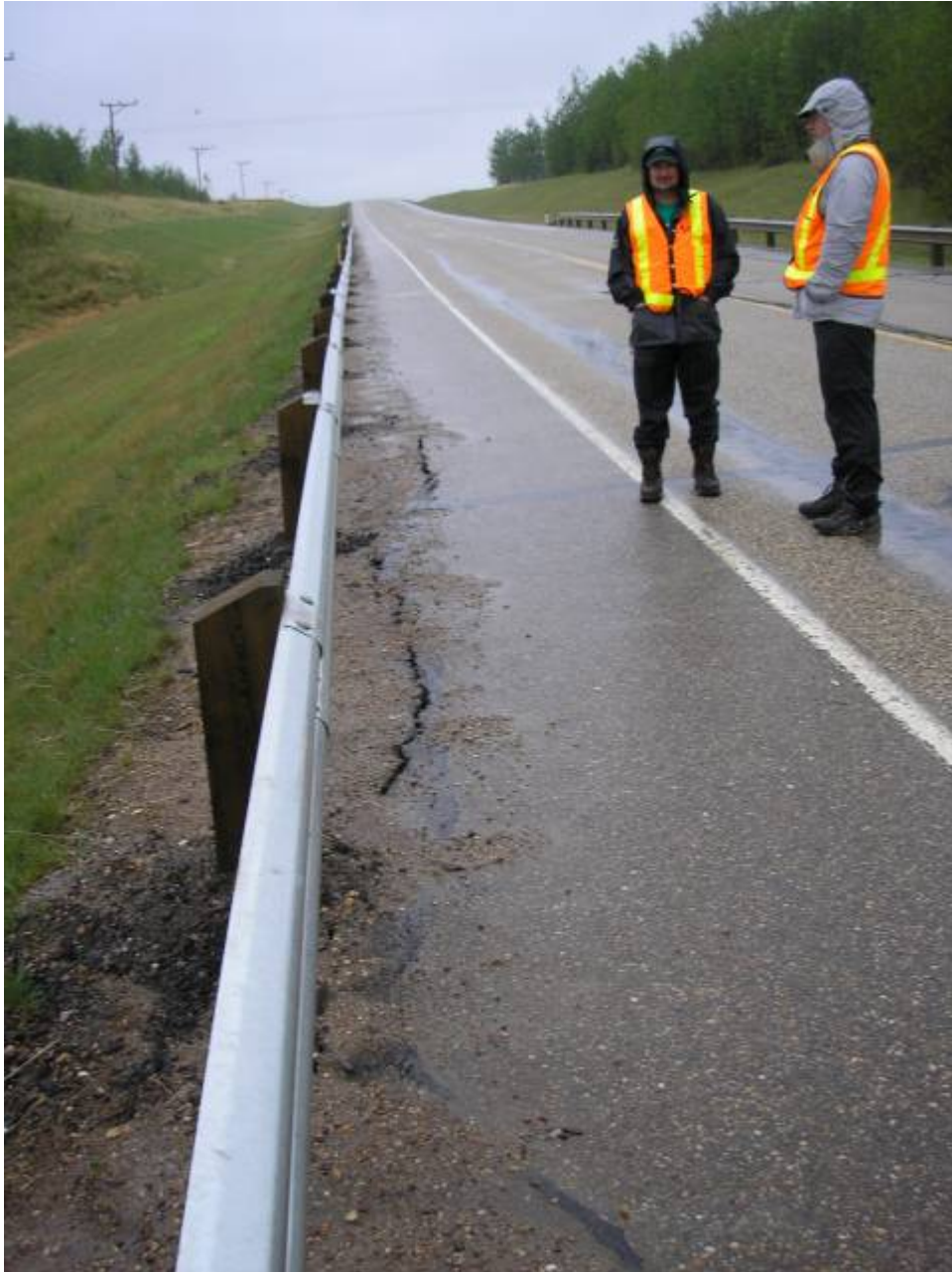
Photo 1 - Looking east along north guardrail, May 25, 2006.
