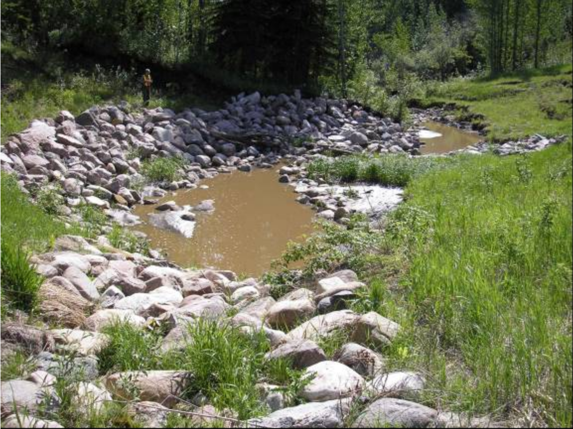
Photo 1 - Looking south along culvert outlet riprap, June 13, 2007.
