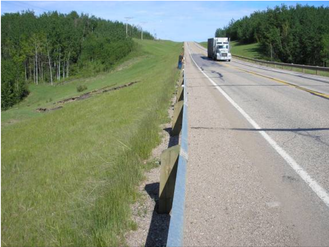
Photo 3 – East view along north guardrail, June 13, 2007.
