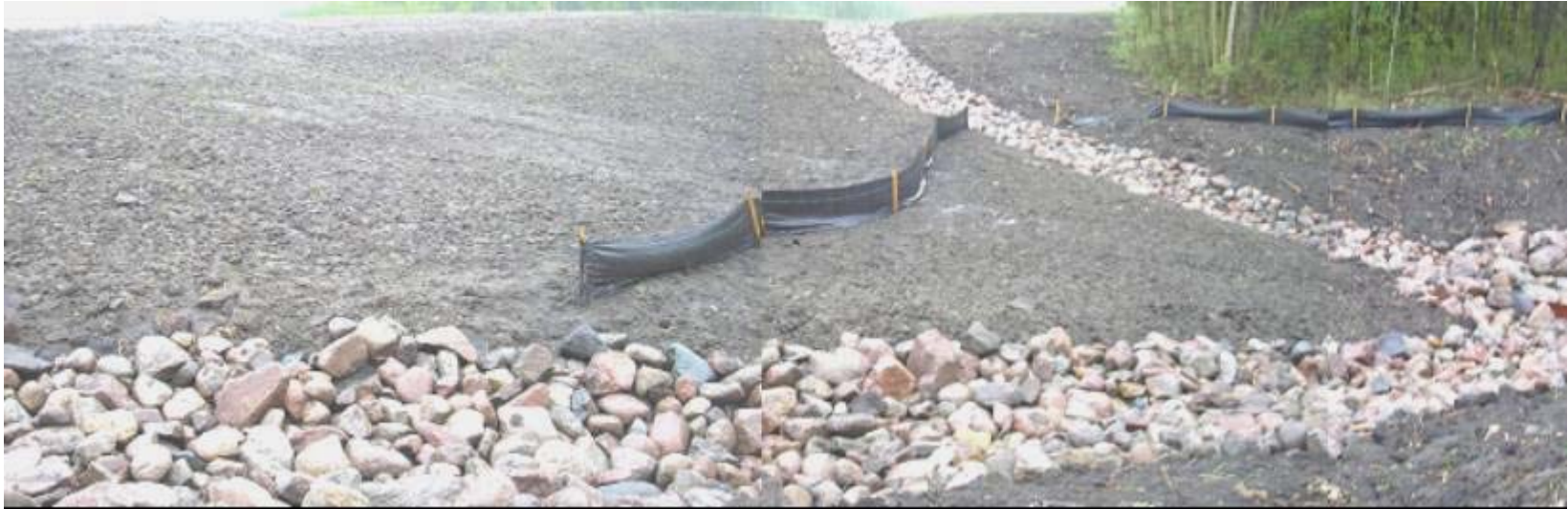
Photo 2 - Looking east at the highway embankment and swale, May 25, 2006.
