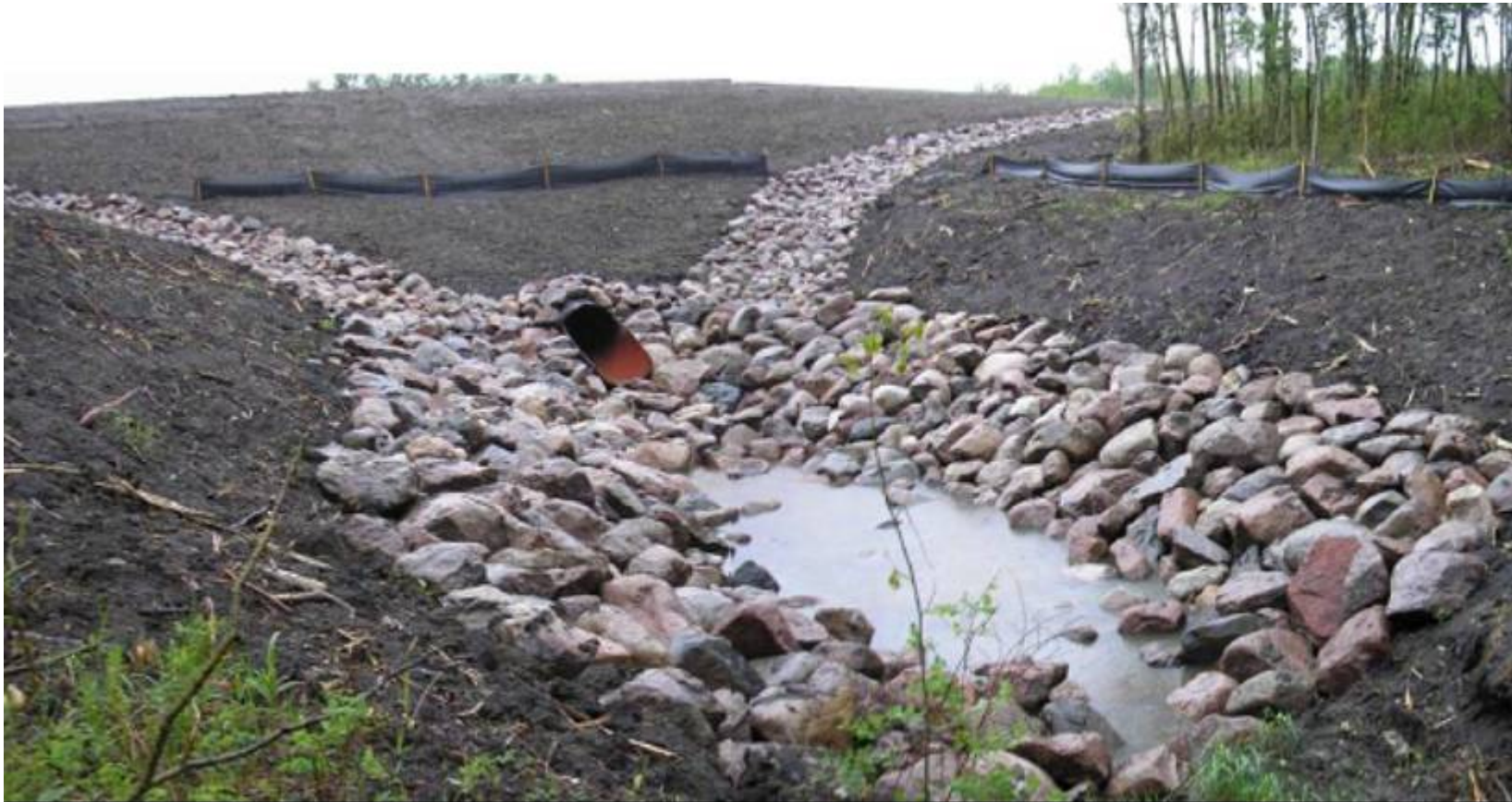
Photo 1 - Looking north at the culvert outlet, swale and reconstructed slope, May 25, 2006.
