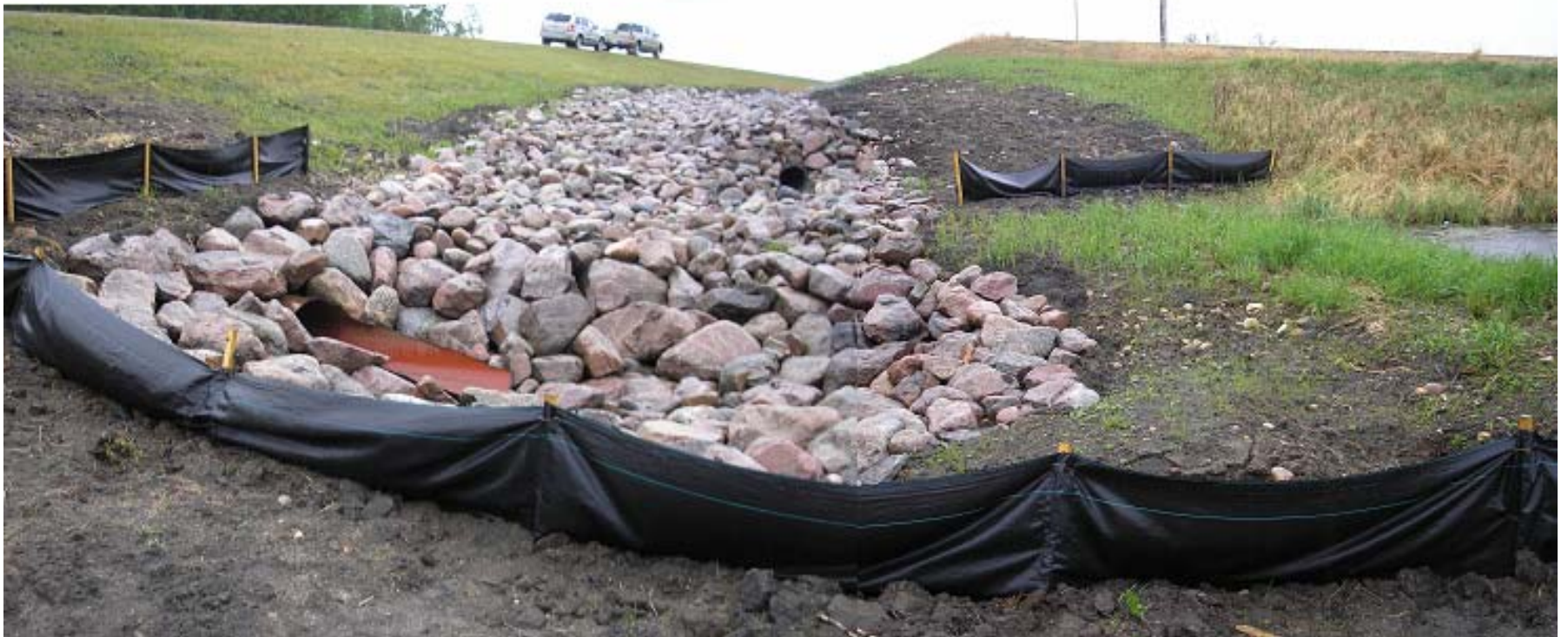
Photo 3 - Looking southwest towards culvert inlet, sub-drain outlet and swale riprap of Site #1A, May 25, 2006.
