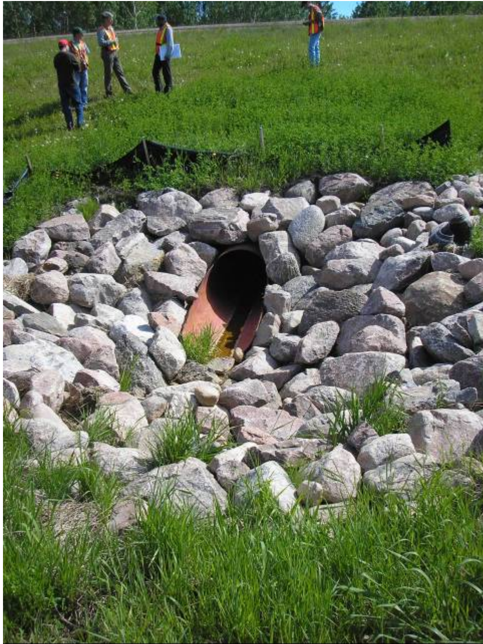
Photo 2 - Looking south at the culvert inlet, June 13, 2007.
