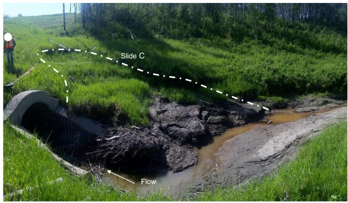
Photo 4: (looking west) Shallow slumping (Slide C) on west bank of Gunns Creek. Fresh toe bulge apparent.
