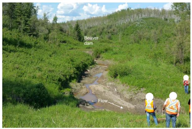
Photo 5: (looking north) Erosion of east and west banks of Gunns Creek adjacent to the culvert inlet. Note beaver dam in background.
