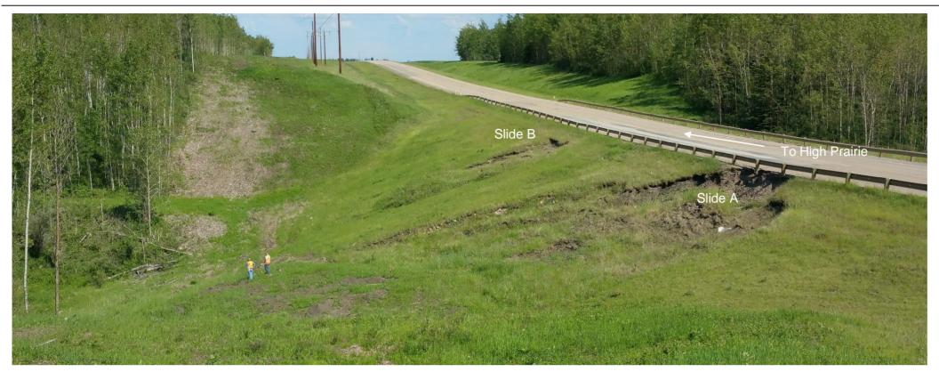
**Photo 1**: (looking east) Overall view of Slides A and B from western approach
