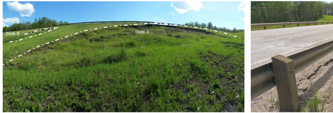
**Photo 2**: (looking south) Slumped mass of Slide A.
