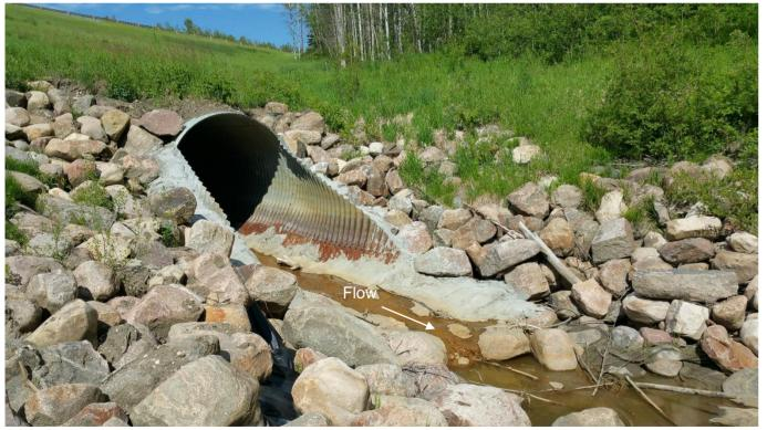
Photo 6: (looking northeast) Geotextile and riprap placed around culvert outlet between 2013 and 2014 inspections. No discernible displacement of riprap has occurred since the 2014 inspection.
