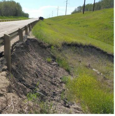
Exposed headscarp of Slide A. Tension cracking near the headscarp of Slide A adjacent to guardrail.
