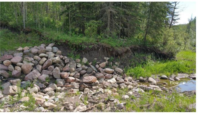
Photo 7: (looking south) Erosion near culvert outlet at south embankment.
