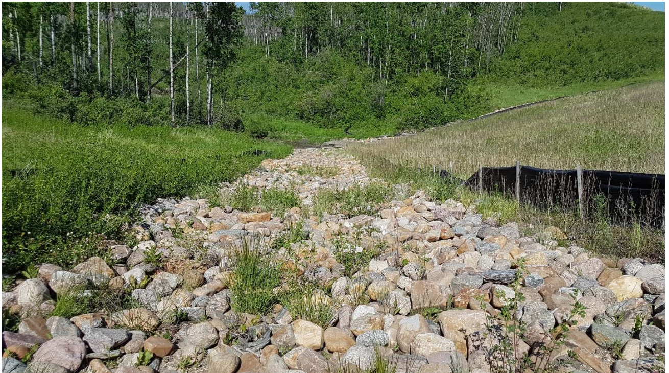
Photo 2 – Looking northeast at riprap-lined ditch channel.
