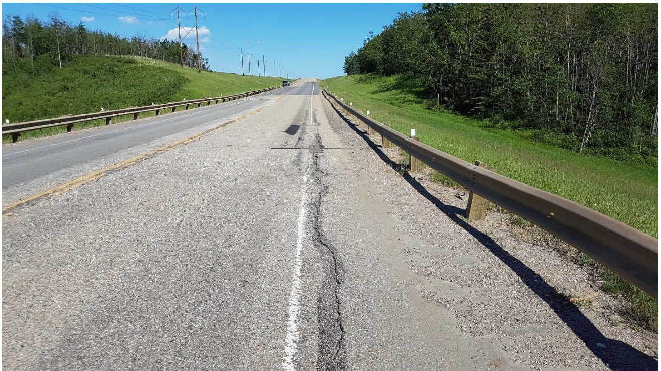
Photo 4 – Looking east at un-overlaid portion of the pavement at this site.
