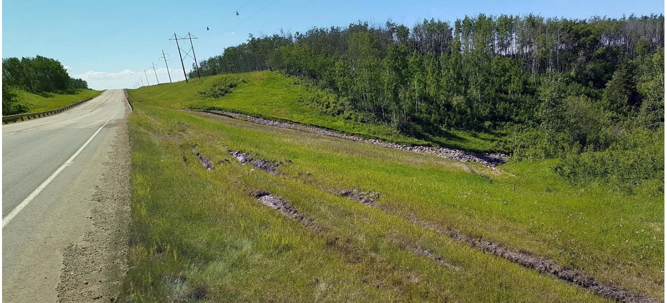
Photo 1 – Looking west at crest of repaired north embankment.
