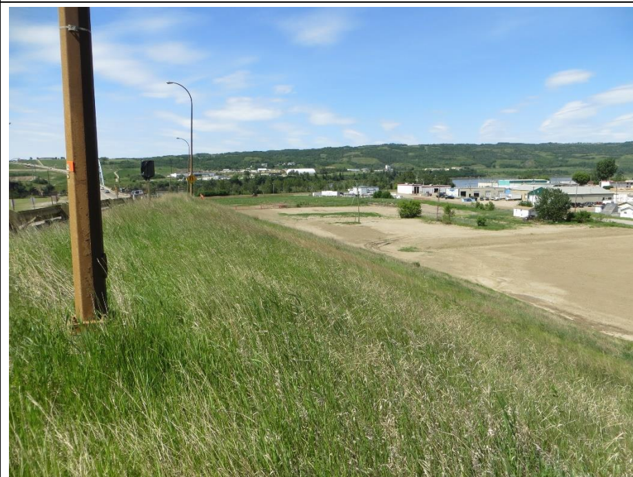
Photo 12. Looking northwest from the 98 Street/Hwy 2:60 on-ramp shoulder towards the former Alberta Transportation yard that has been regraded as part of the salt contamination remediation in the spring of 2017.
