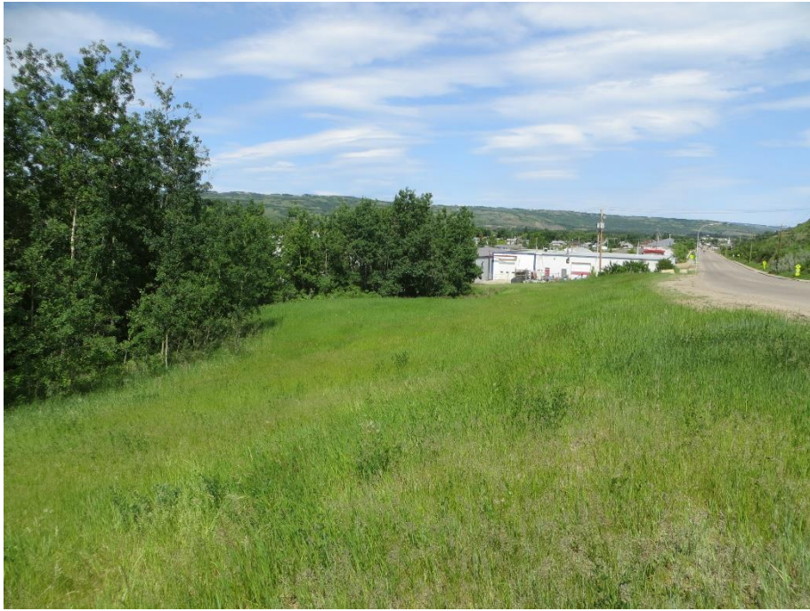
Photo 1. Looking north along the top of bank west of 98 Street north of the Hwy 2:60 on-ramp. There is a distinct dip in the sideslope at the top of bank.
