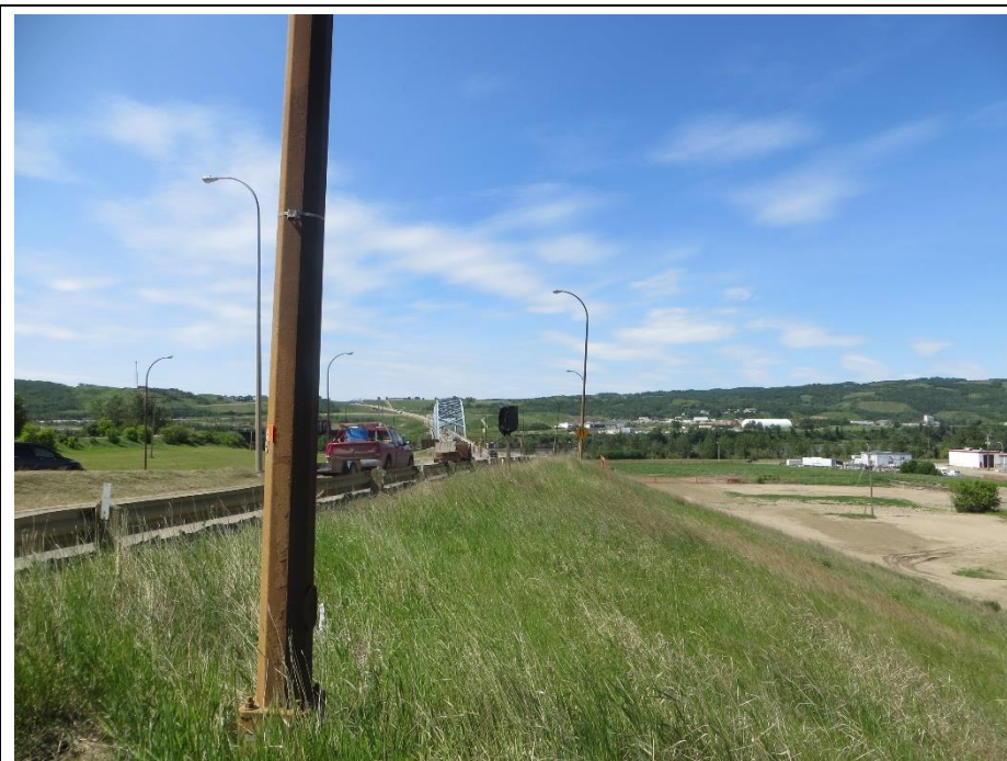
Photo 13. Looking west along the sideslope of the 98 Street/Hwy 2:60 on-ramp. The embankment is about 13m in height
