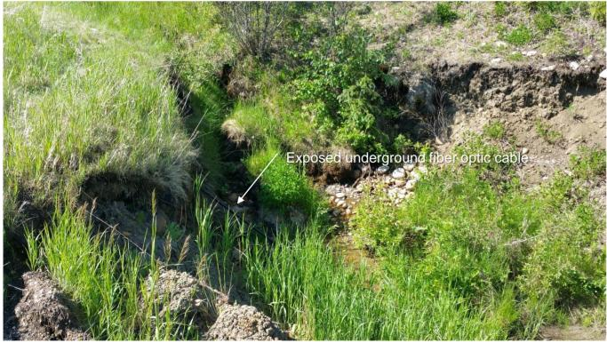
Photo 3: (looking east) Note depth of erosion gully, erosion of highway embankment fill, and exposed cable.
