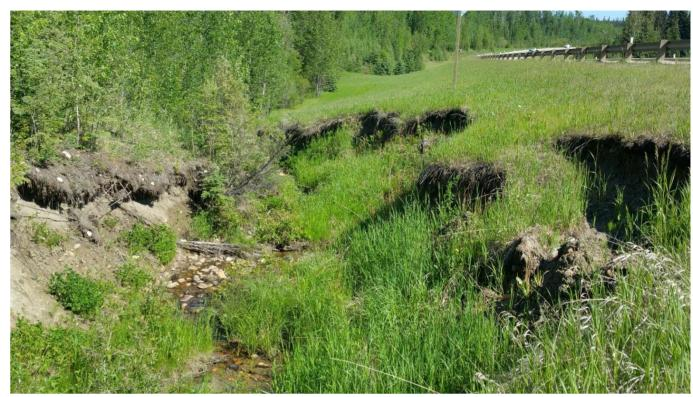
Photo 2: (looking north) Note depth of erosion gully and erosion of highway embankment fill.
