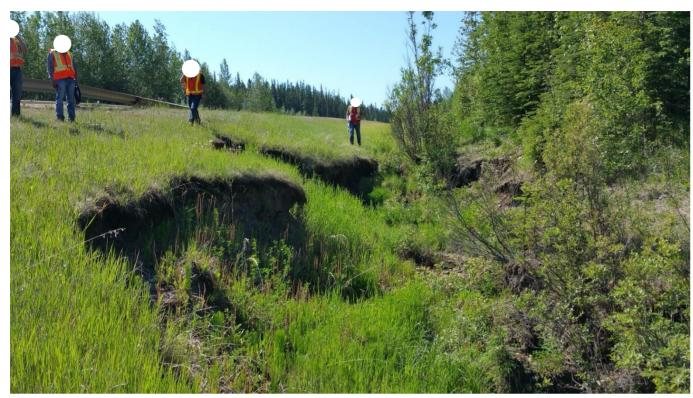
Photo 1: (looking south) Erosion and slumping in west ditch of Highway 32. Erosion gully was approximately ~5.7 m from the white line of the highway.
