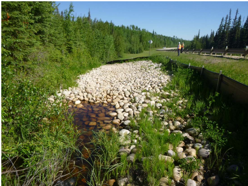
Photo 6 – Looking north at regraded and lined SH027A gully area.
