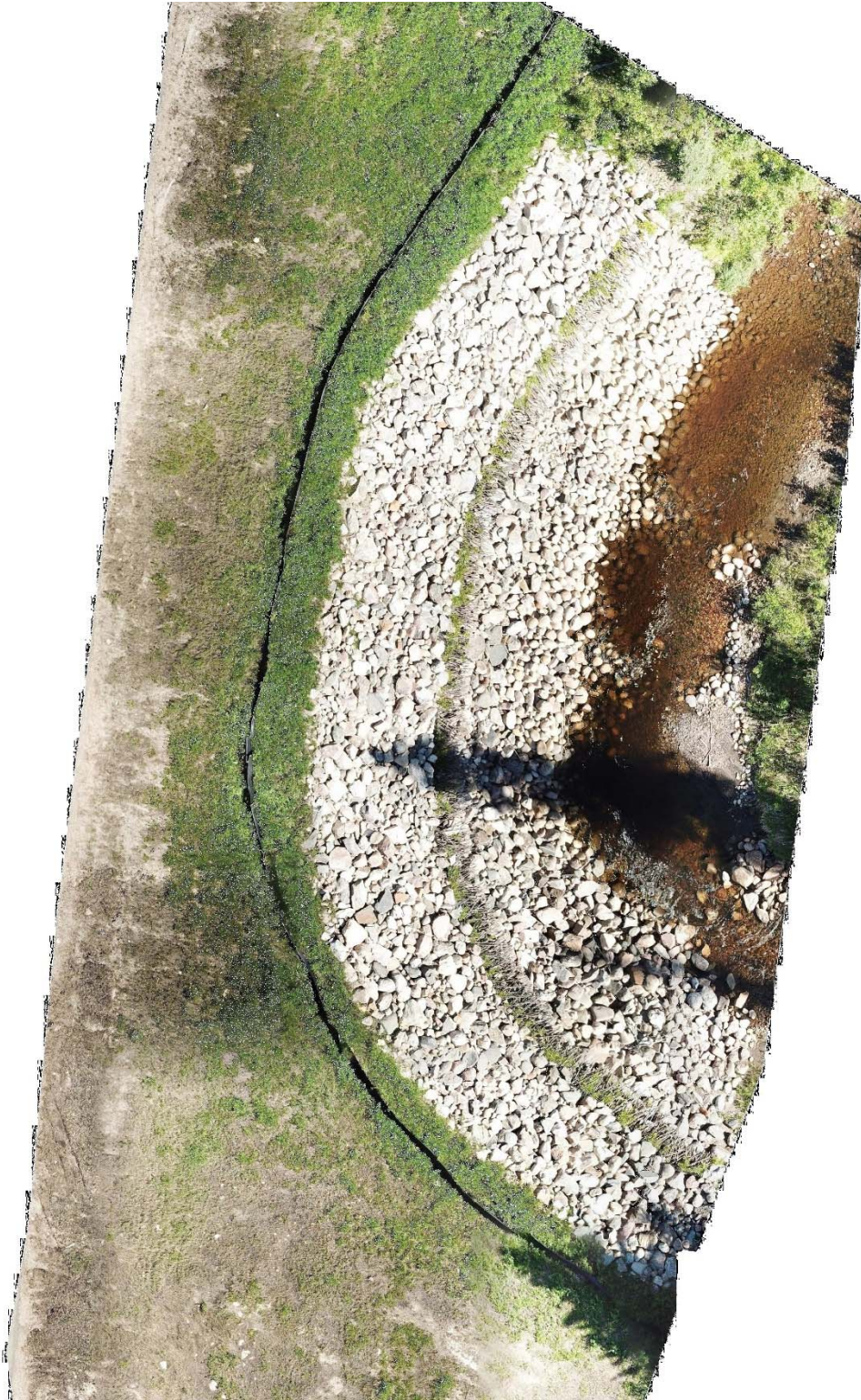
UAV Composite Image of Rebuilt Area
