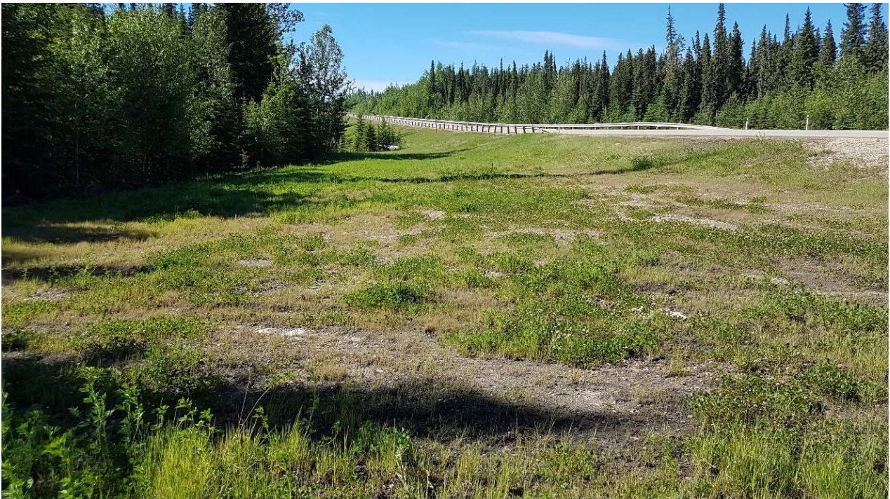
Photo 4 – Looking south at sparser growth in construction laydown area south of realigned channel area.
