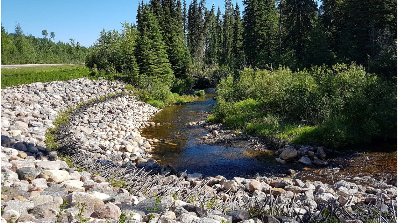
Photo 1 – Looking north at realigned channel.
