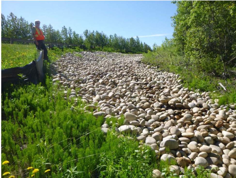
Photo 5 – Looking south at regraded and lined SH027A gully area.
