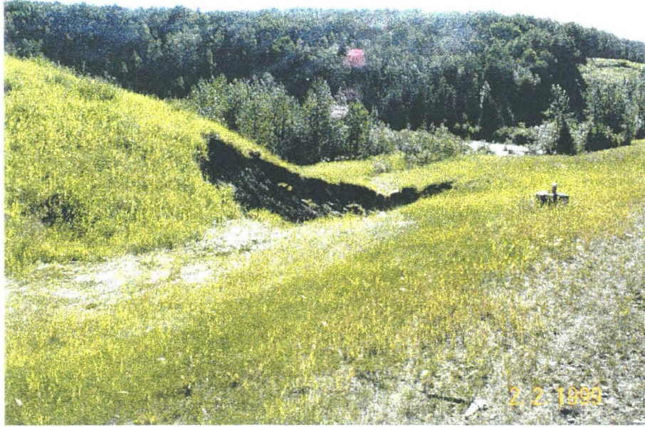
VIEW OF ERODED EMBANKMENT SECTION LOOKING EAST
