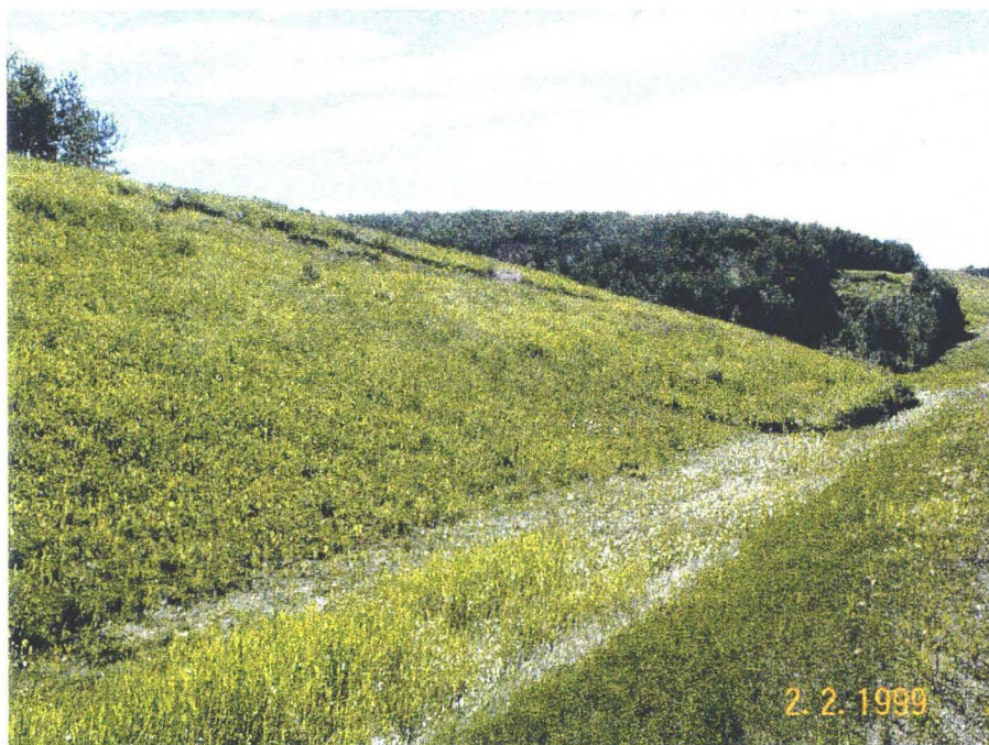
VIEW OF NORTH EMBANKMENT SLIDE AREA LOOKING EAST
