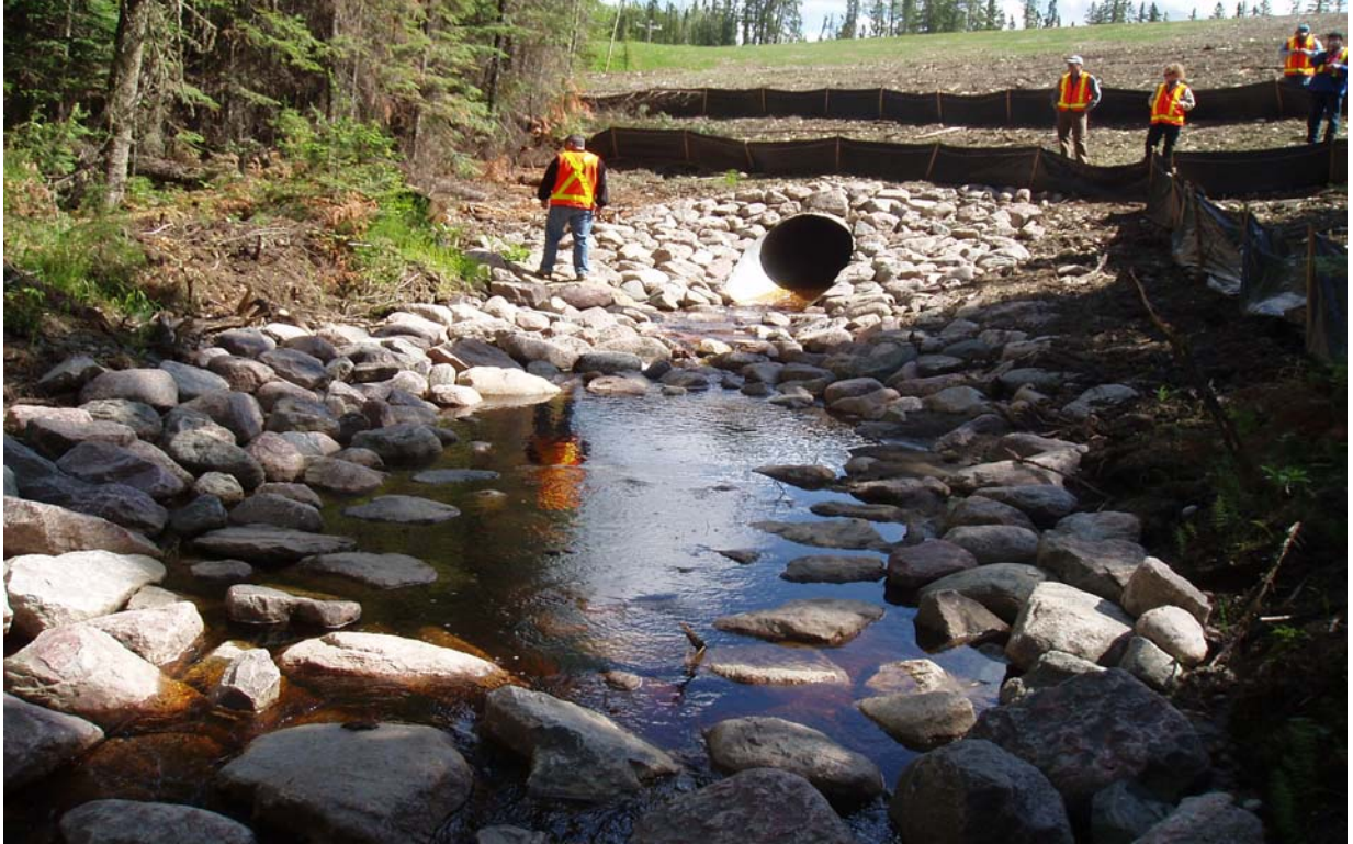
Photo 2: Looking northeast at culvert outlet. Note loose silt fence south of creek.
