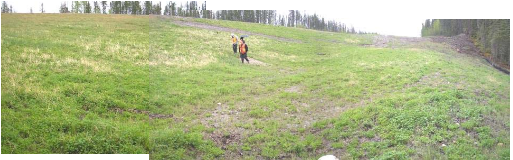
Photo 1 - Looking south to southwest along slope and culvert outlet, May 23, 2006.
