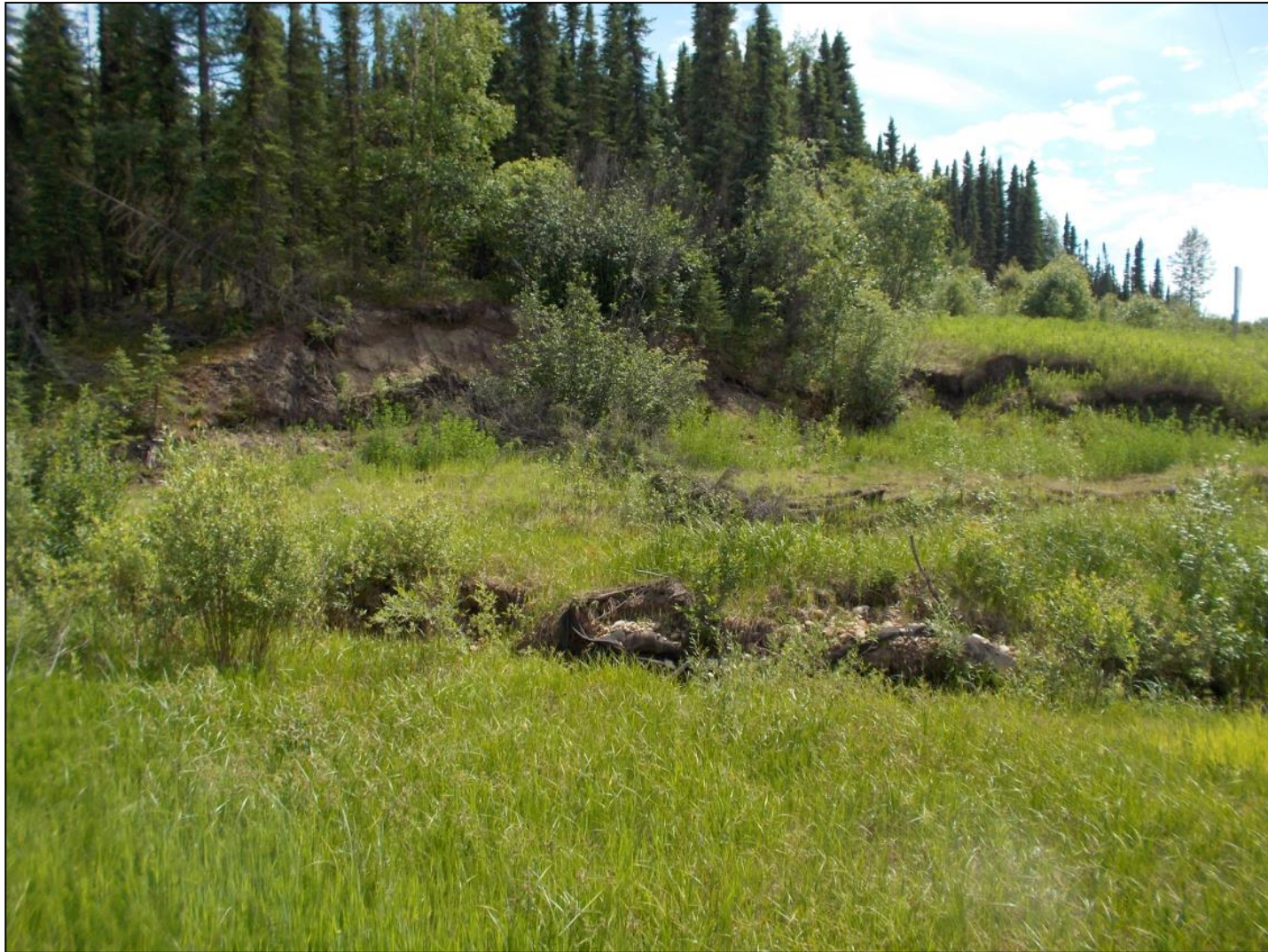
Photo 1: Slumping of slope looking south from Deer Mountain Road. Failed biowall within main body of slide visible in centre/centre right of photo.
