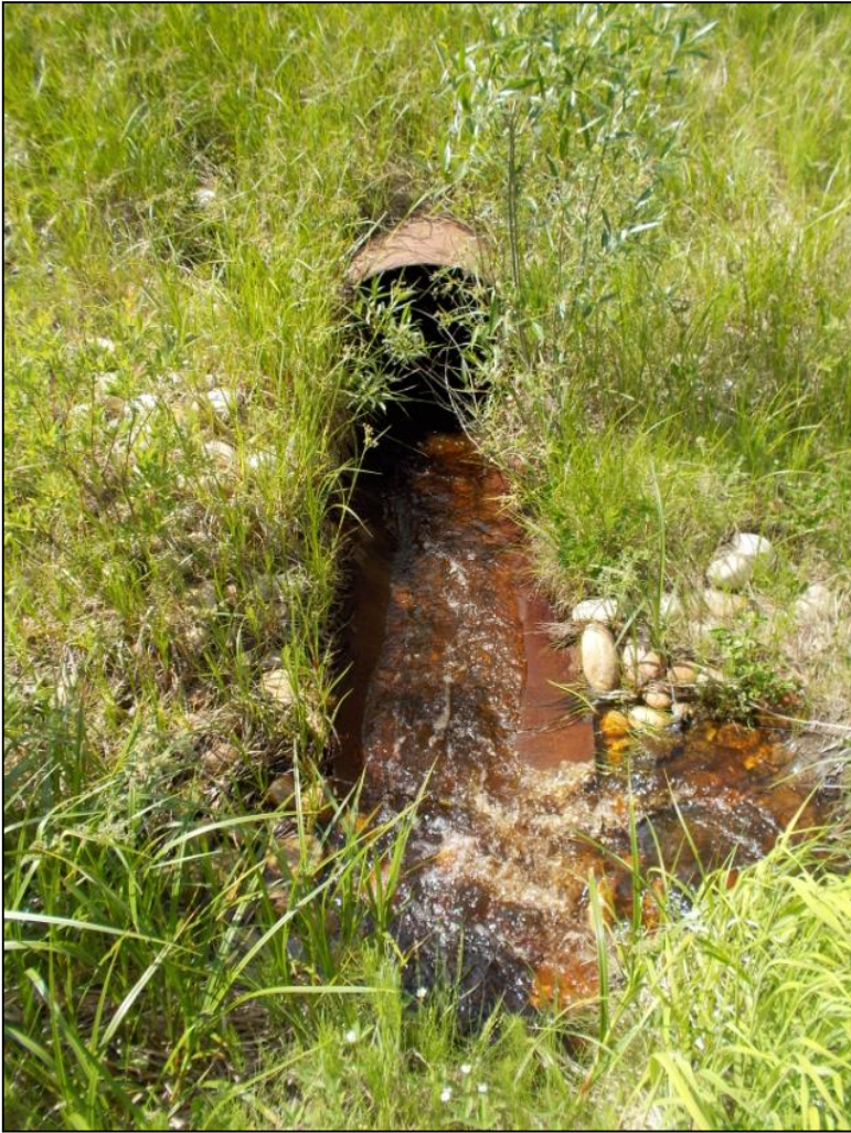
Photo 2: Culvert inlet east of Highway 33
