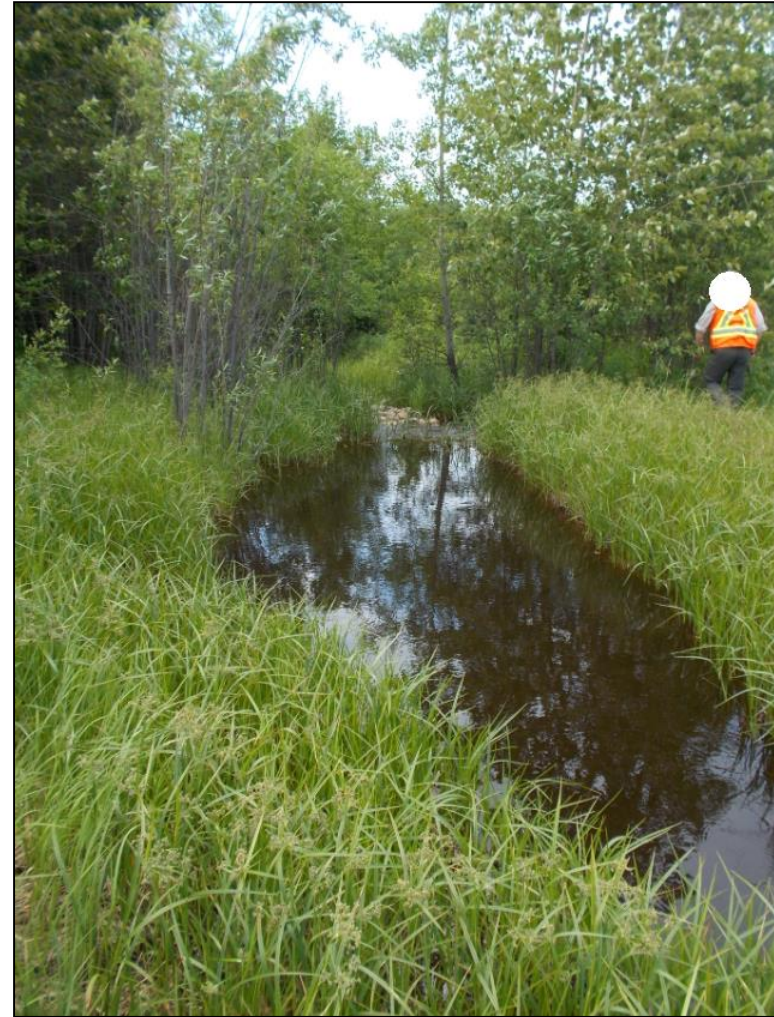
Photo 3: Looking west at pond downstream of culvert outlet west of Highway 33. Culvert outlet (not visible) below water at bottom of picture
