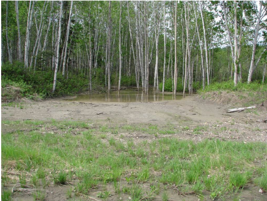
Photo 5 – Silt sediments accumulated near the toe of the slope, looking northwest.
