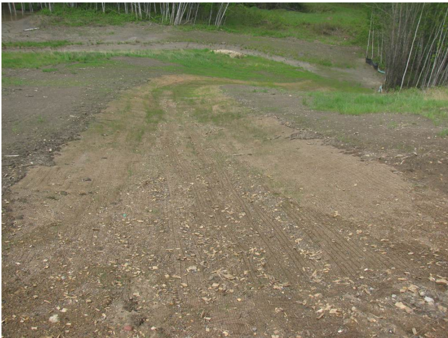
Photo 6 – Drainage swale on the east side of slope, looking northwest.
