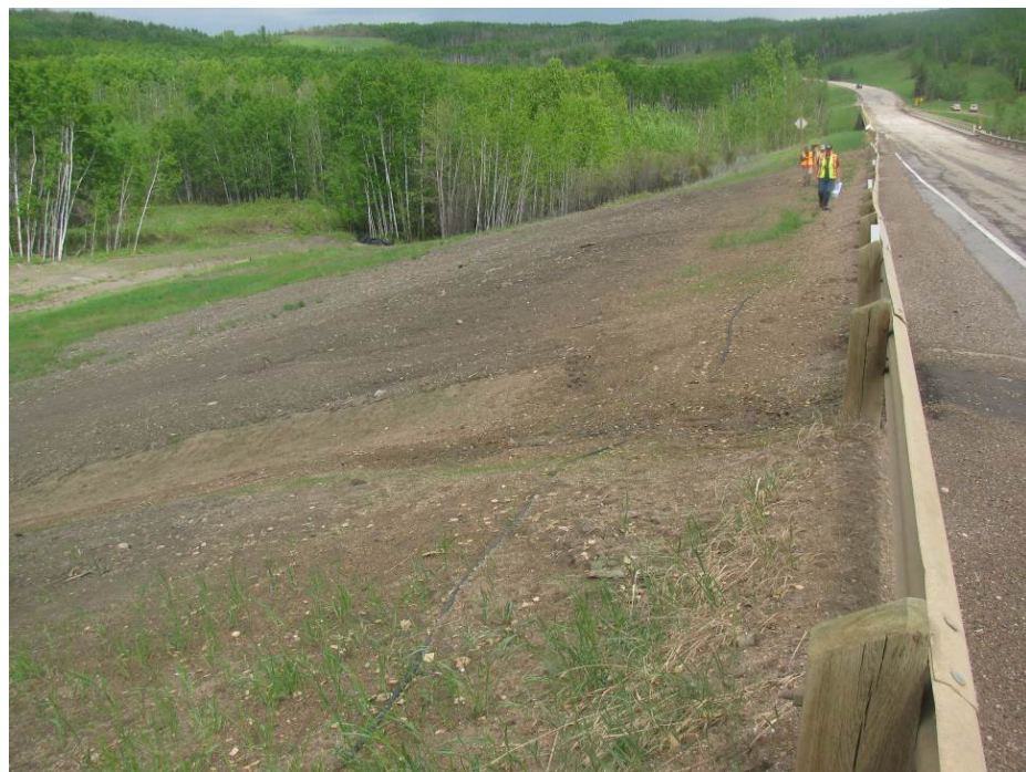
Photo 2 – Side slope and highway, looking northeast.
