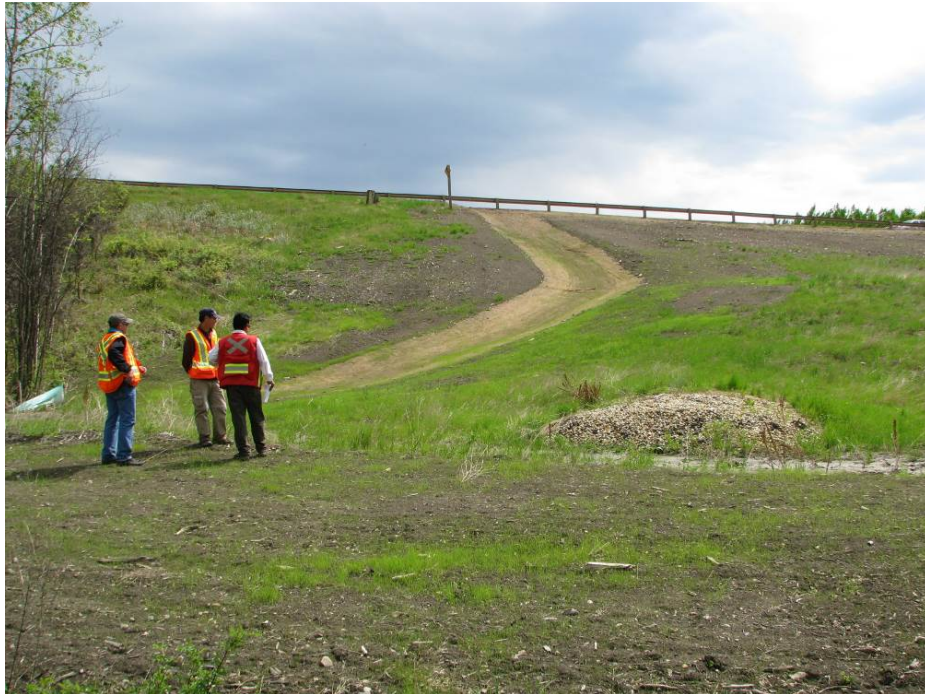
Photo 3 – Side slope and drainage swale, looking southeast.
