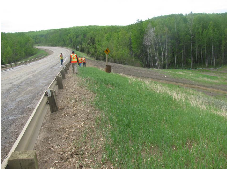
Photo 1 – Side slope and highway, looking southwest.
