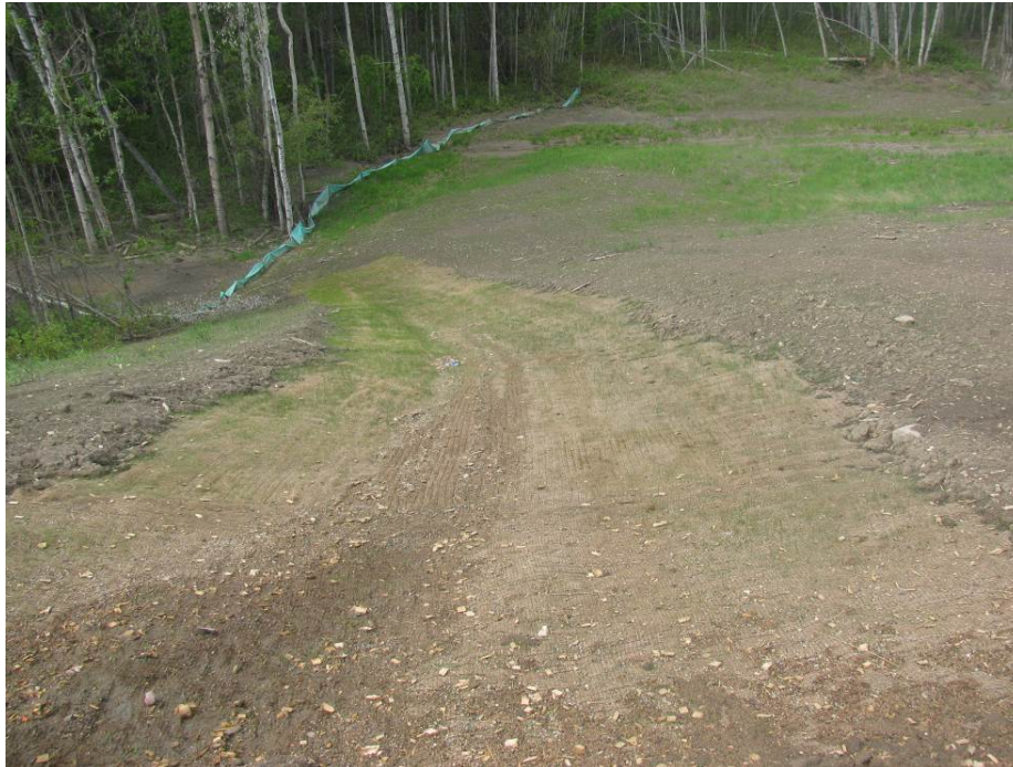
Photo 7 – Drainage swale on the west side of slope, looking northwest.
