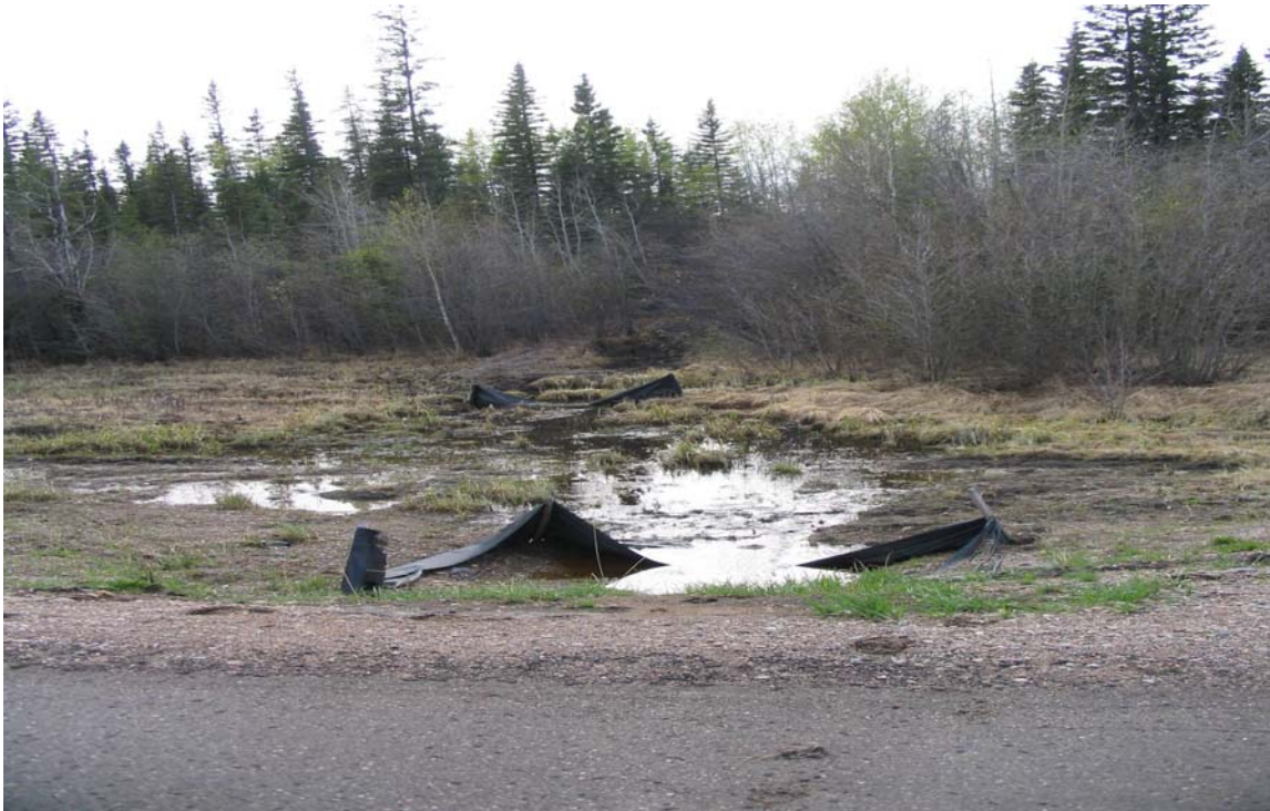
PHOTO 3: Creek and ponded area on west side of highway at Site A.
