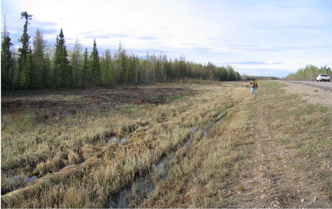
PHOTO 7: Muskeg heave and stagnant water on west side of the highway at Site B.
