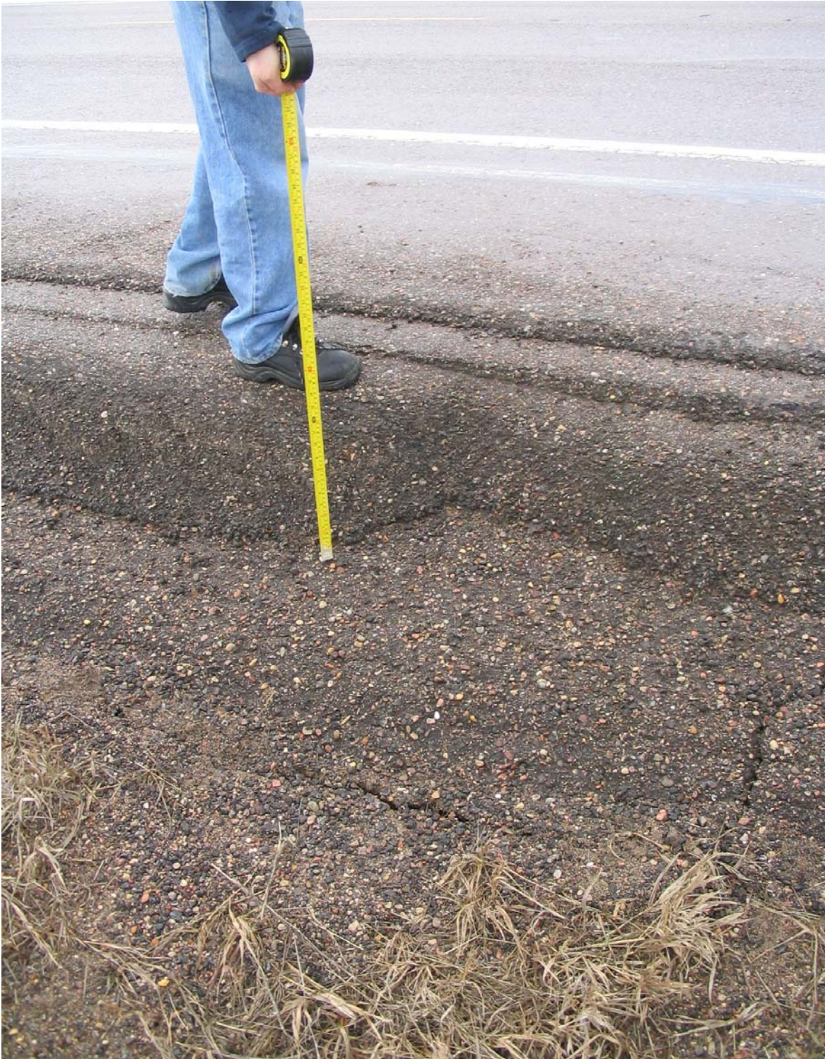
Photo 3 - Overlay 300 mm thick in ACP patch in Site A.
