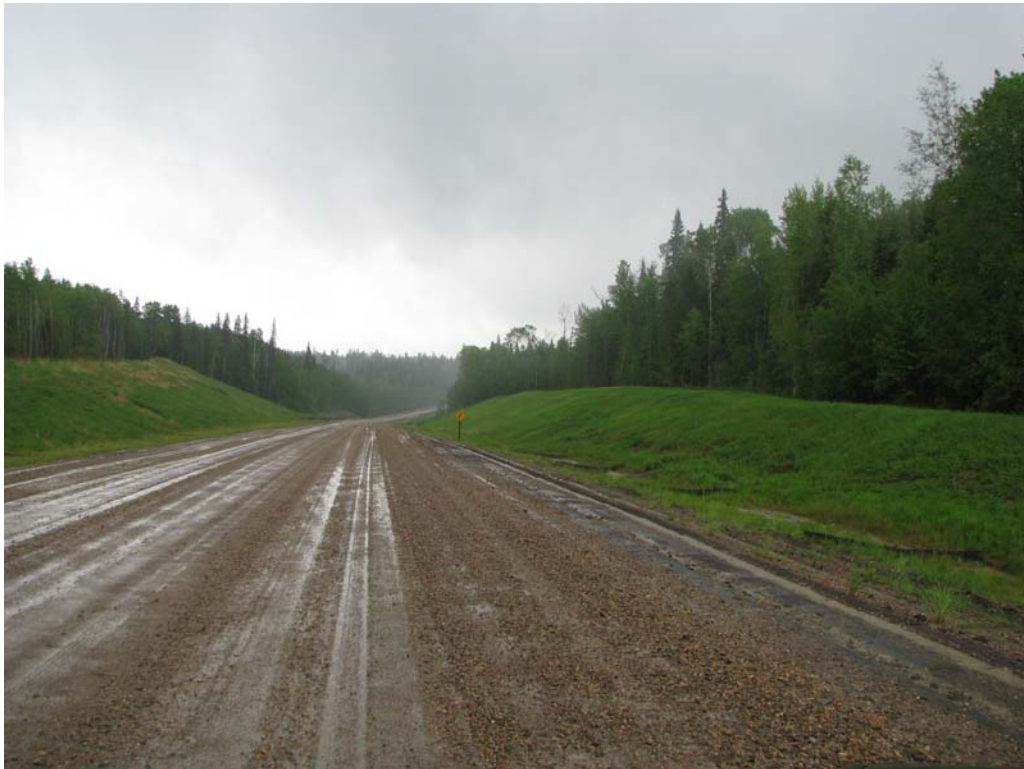
Photo 1 – View of the site showing east and west backslopes, looking southeast.
