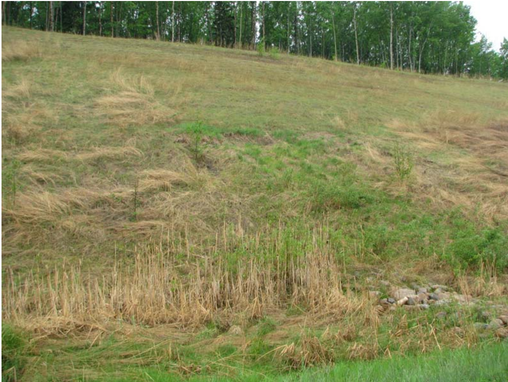
Photo 2 - View of active cracks east of main slump, looking south.
