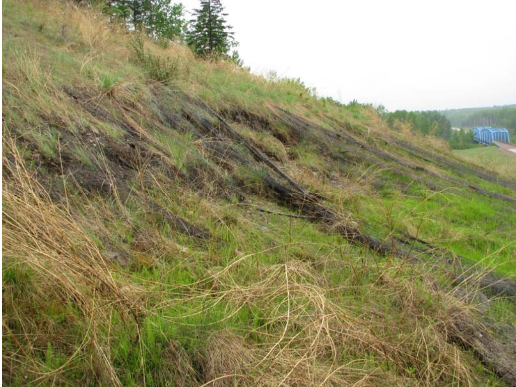
Photo 3 - View of backslope, looking west.
