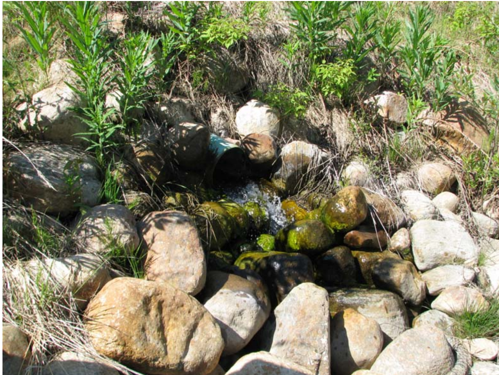
Photo 5 – Fast flow through subdrain, looking southwest.
