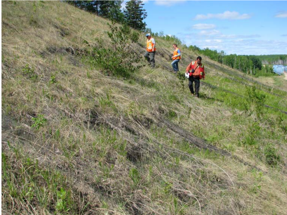
Photo 3 - View of backslope, looking west.
