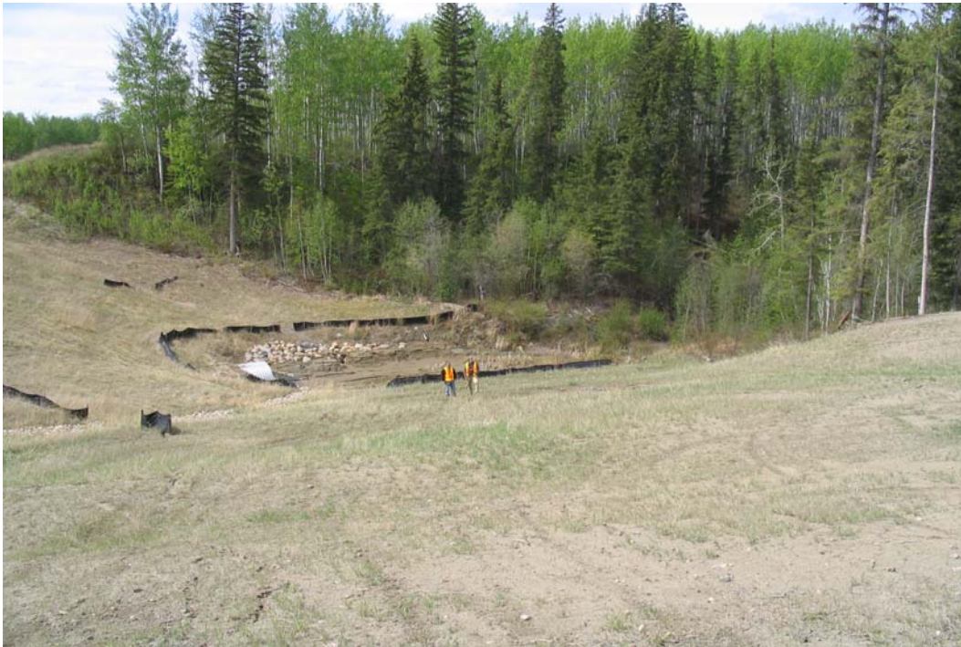
PHOTO 1: Overall view of the west slope.
