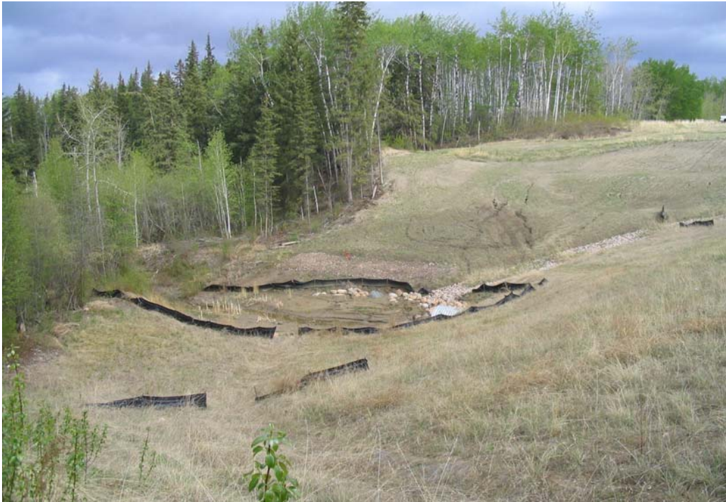
PHOTO 5: Overall view of the east slope.
