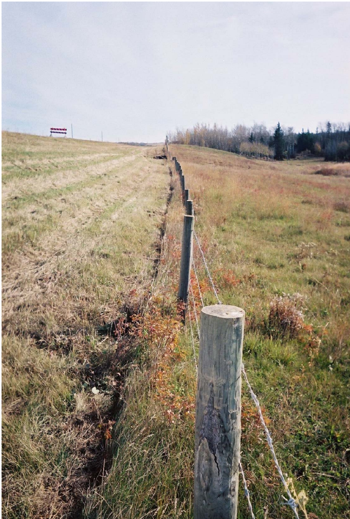
PHOTO 1 - LOOKING EAST ALONG FENCELINE ACROSS SLIDE AREA NOTE SLIGHTLY BOWED FENCE
