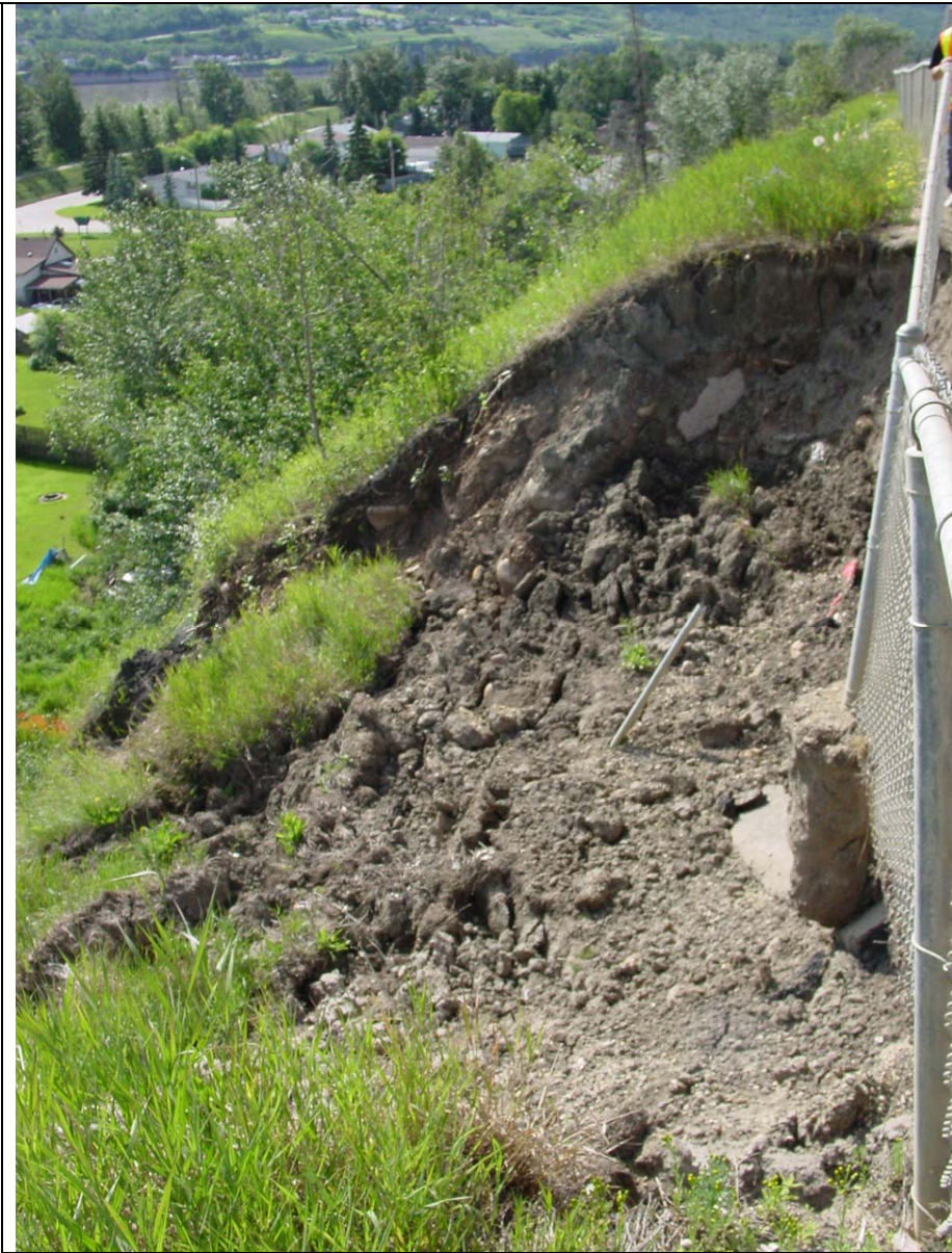
Photo 3. Debris in slide area.
