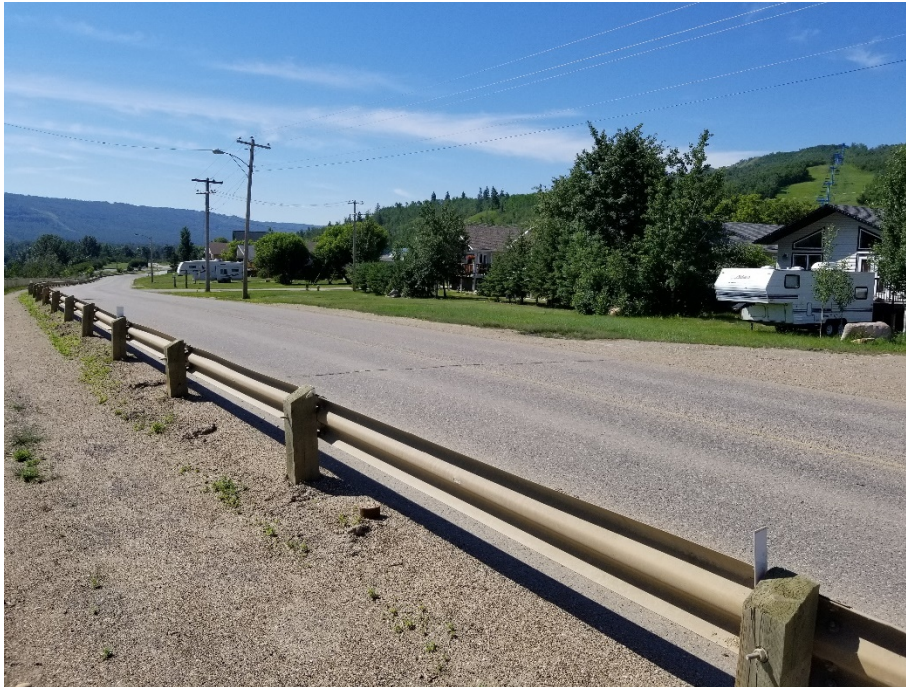
Photo 1: Looking SW at HWY 684 from the NE side of the intersection with 105 Avenue.
