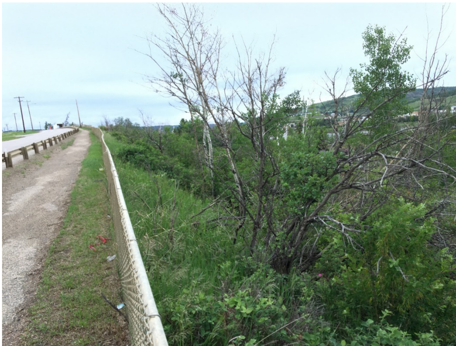
Photo 2: Looking N at the dip in the ACP trail and the bend in the fence above the slide.
