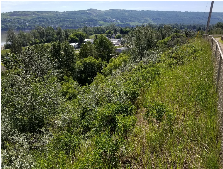
Photo 4: Looking southeast from chain link fence at the landslide
