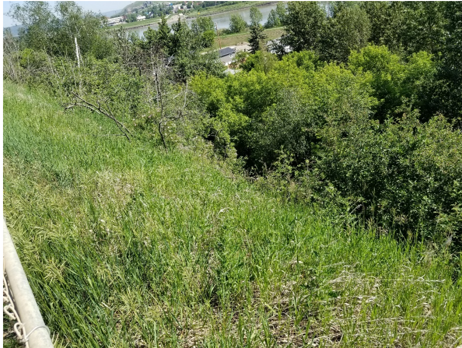
Photo 5: Looking northeast from chain link fence at the landslide
