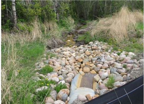
Photo 8. Looking southeast at Bogey landslide culvert outlet rip rap.
