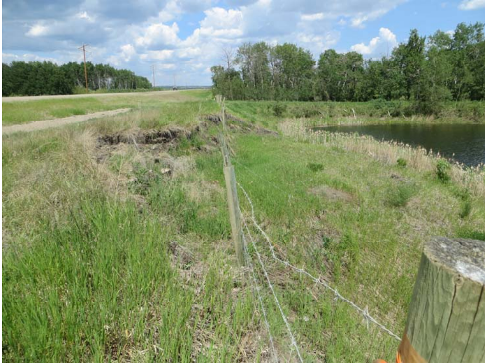
Photo 1 – Looking north at the backscarp of the pond slope failure of the Double Bogey Slide. Hwy 743 is on the left side of the photo.
