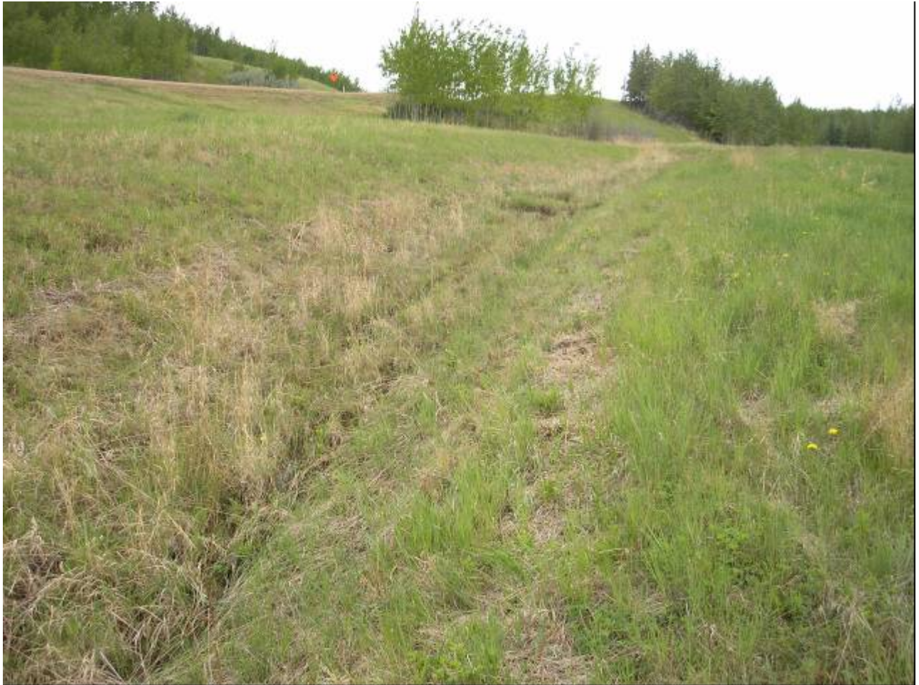
Photo 3 - Looking southwest at rutted ditch area with ponded water, May 24, 2006.
